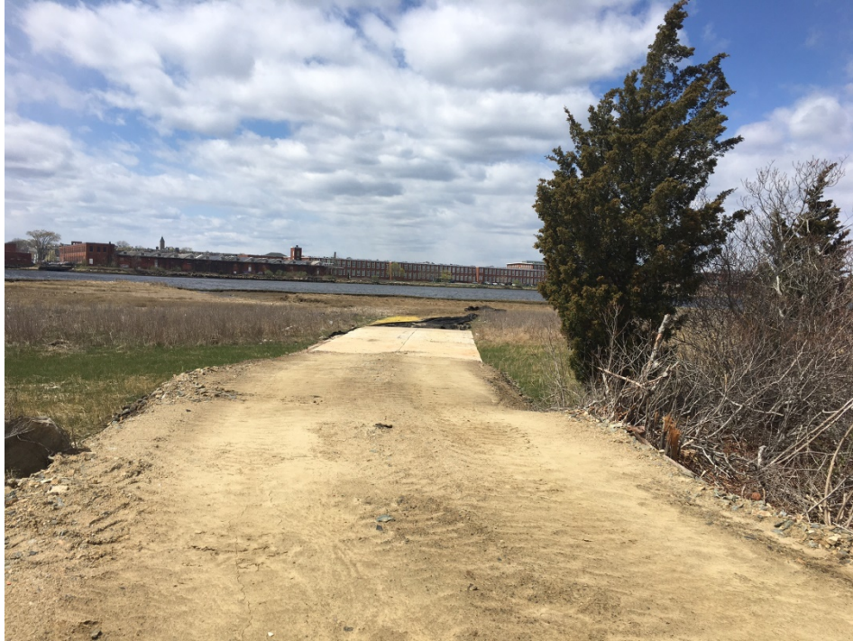
Typical haul road branch through TRANSITION ZONE and HIGH TIDE BUSH ZONE
