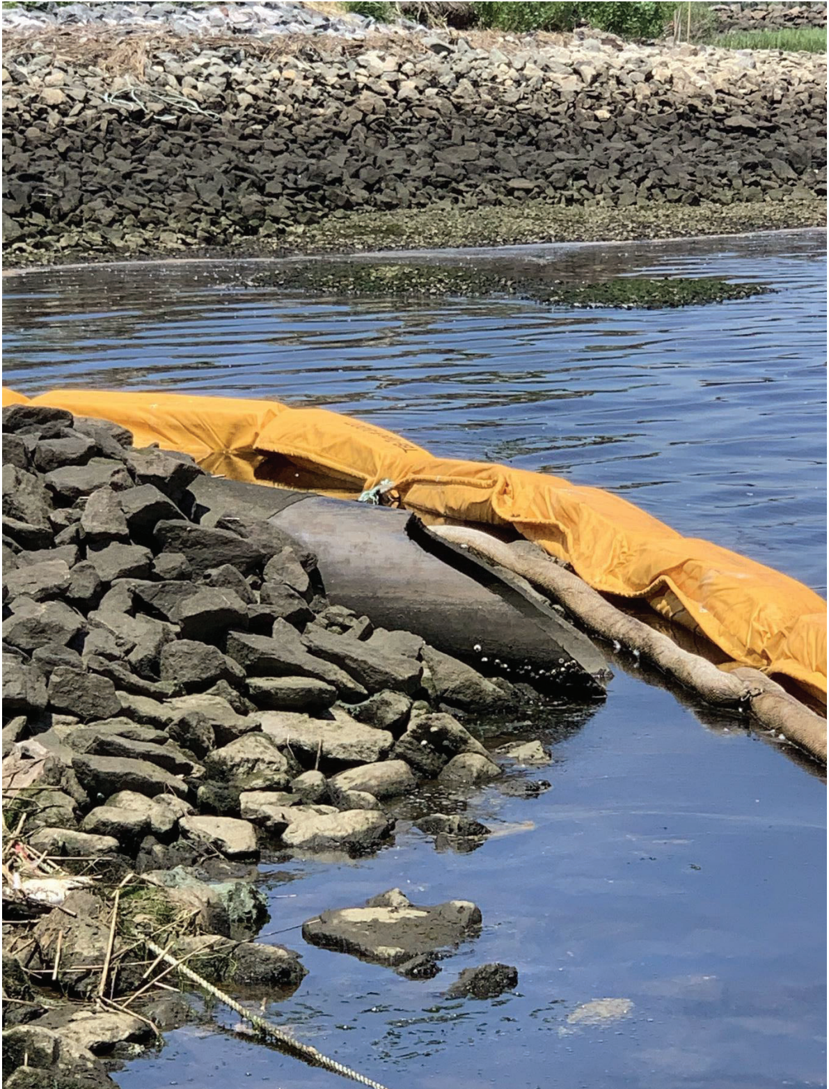
Photo #4: This photo shows the discharge/seaward end of the north trench stormwater pipe; view looking north (the northern bank of the sediment cap is in the background).
