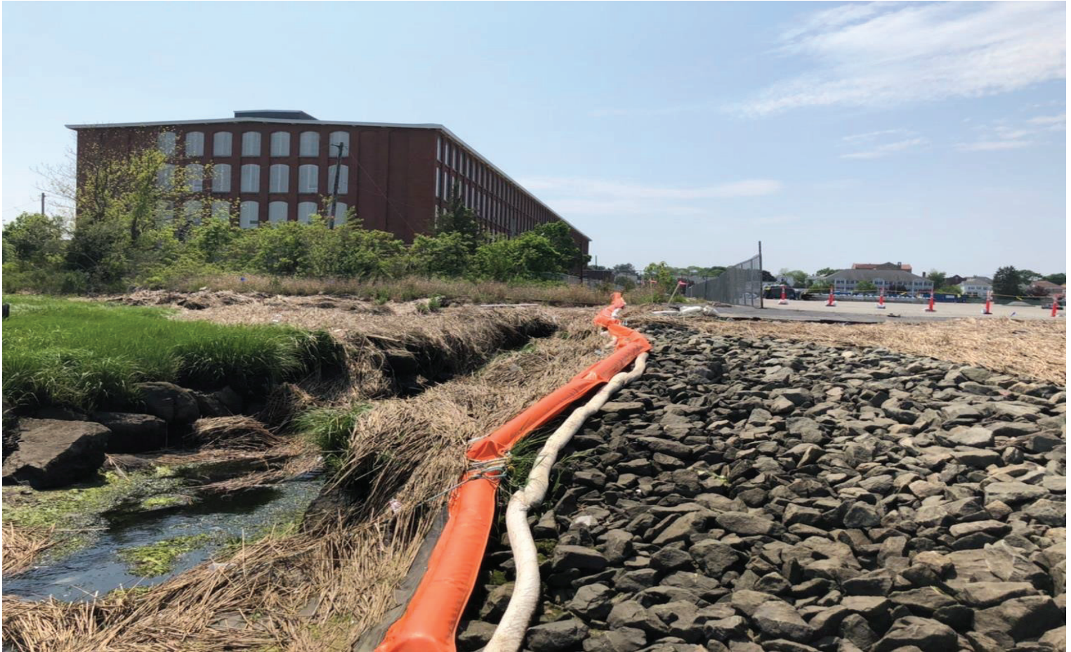
Photo #10: Looking west along the southern edge of the sediment cap. City storm drain outfall to the left; Titleist facility in background. Note marine rack line at the top of the stone bank as well as along the 21E silt curtain.
