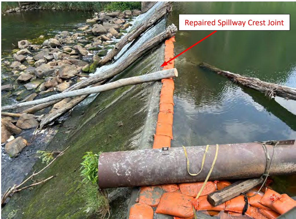
Photo 6. Spillway crest joint after repairs.
