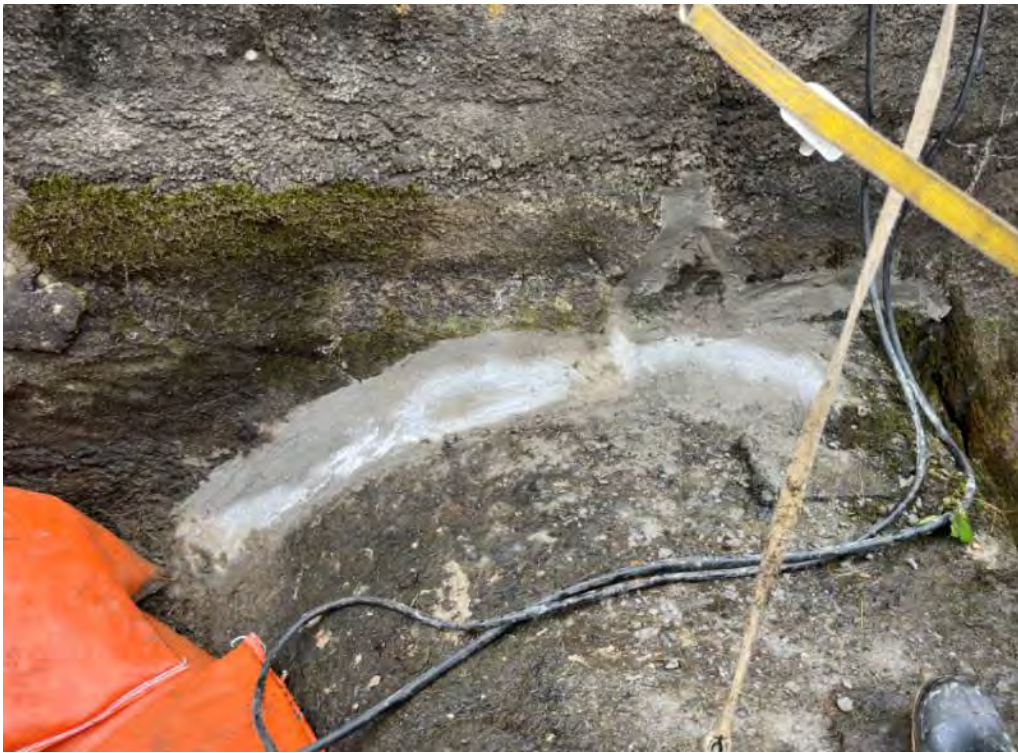
Photo 4. Former vortex repair area after repairs.
