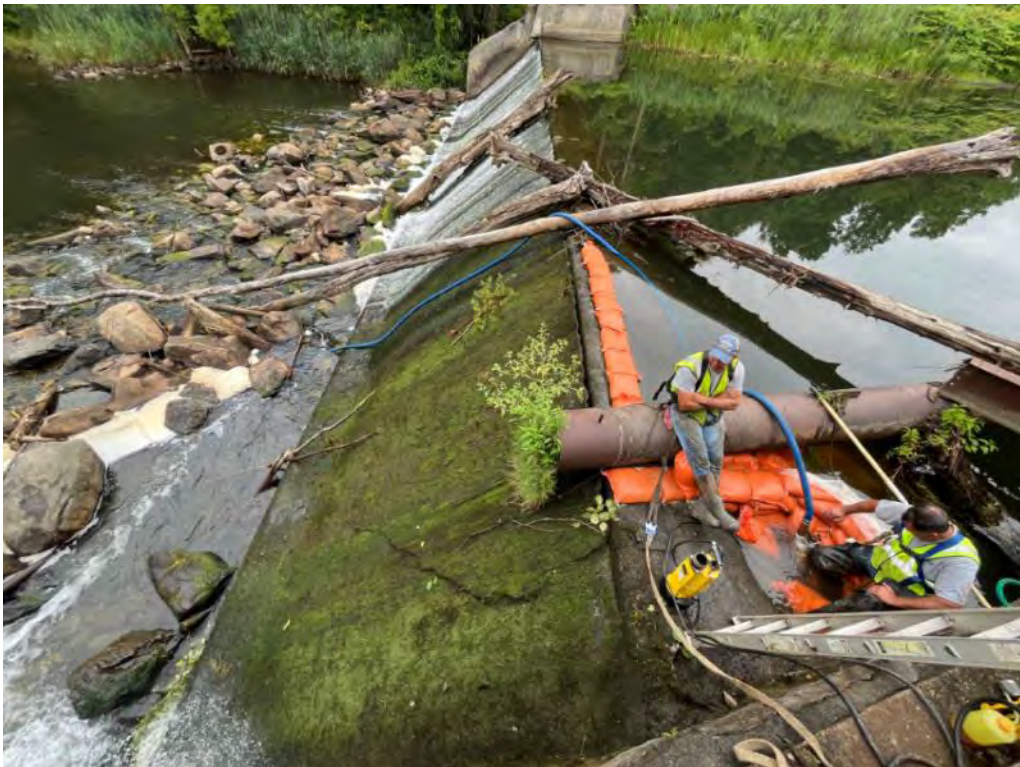
Photo 2. Temporary sandbag cofferdam installed. Installing dewatering pumps.
