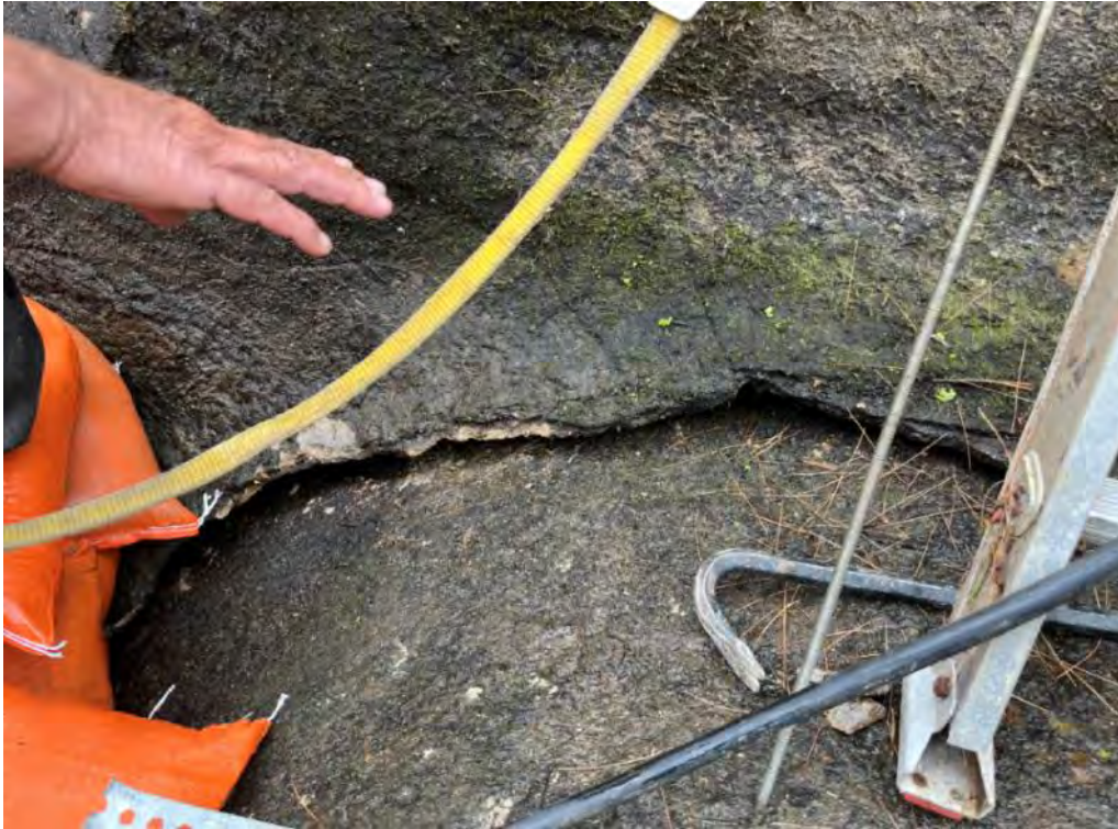
Photo 3. Former vortex repair area prior to repairs.
