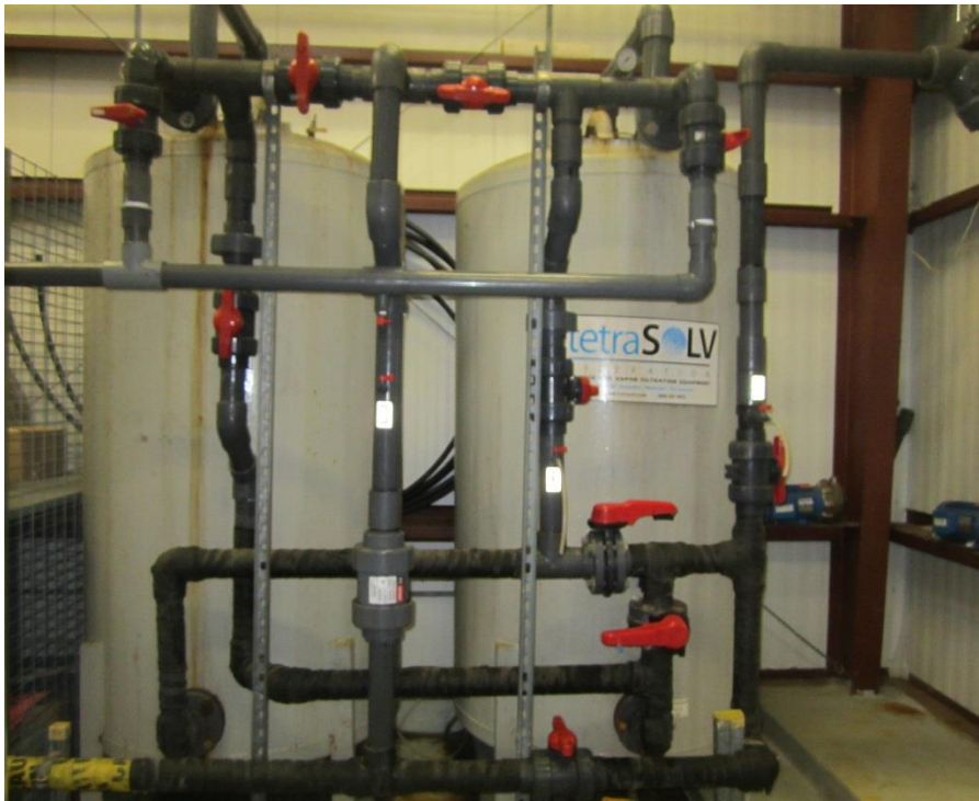
Photo 4. T-25 Treatment System 2,000 lbs. liquid phase carbon vessels.
