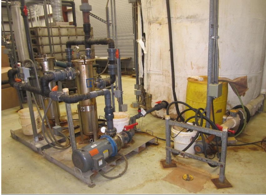
Photo 3. T-25 Treatment System equalization tank, bag filters and influent sampling port.
