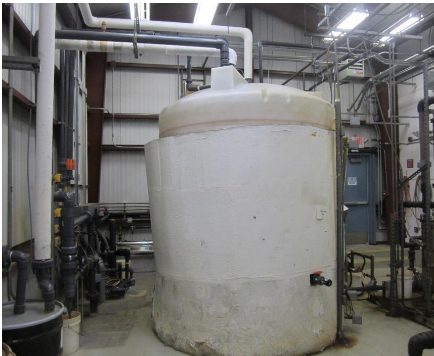
Photo 2. T-25 Treatment System. Pipes from extraction wells entering into equalization tank.
