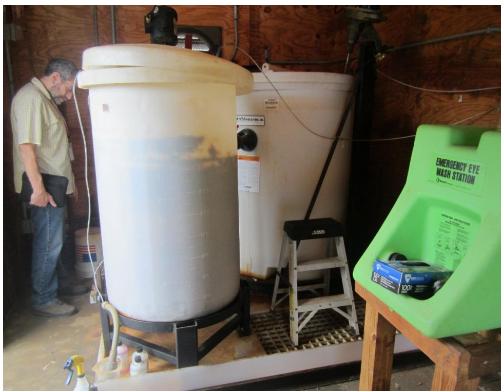
Photo 8. 1,4-Dioxane pre-treatment unit mixing and reactant tanks.
