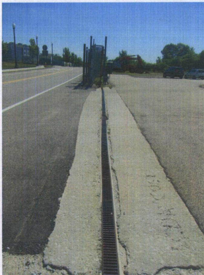
Photograph 4: Polydrain at Facility Entrance from Catch Basin CB-3
