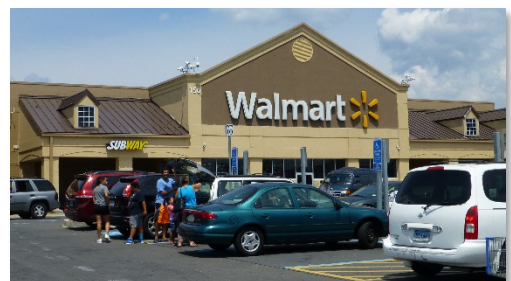
Figure 5. Views of the Home Depot and Walmart at the Stratford Crossing Shopping Center.
