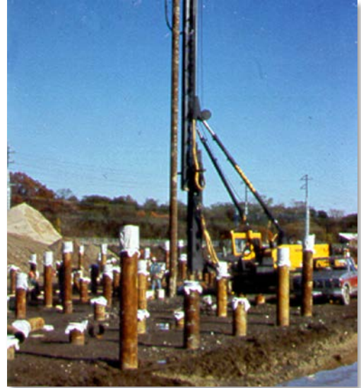
Figure 4. Subsurface work prepared the site for future commercial use.
