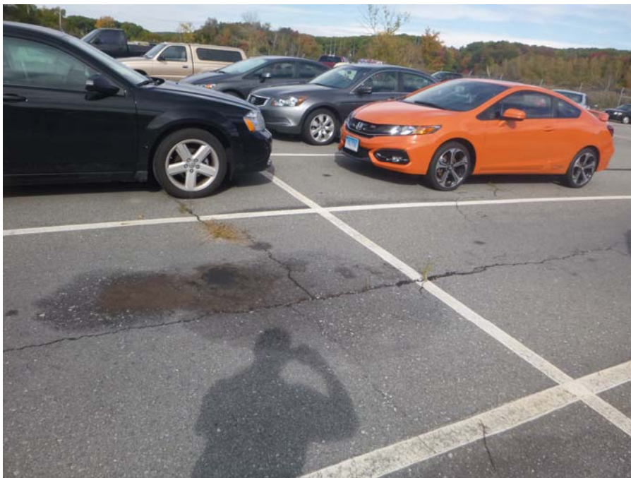
2A-3 Site 2A – Area A Landfill Deployed Parking Area Typical cracks
