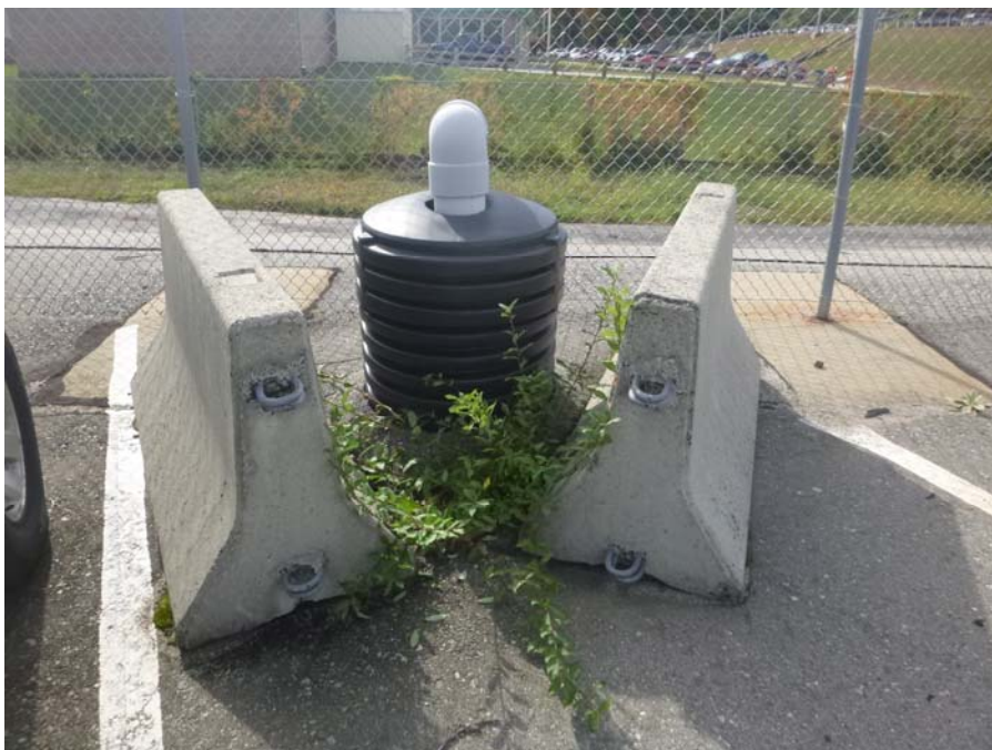
2A-4 Site 2A – Area A Landfill Deployed Parking Area Cracks with vegetation located near a landfill gas vent
