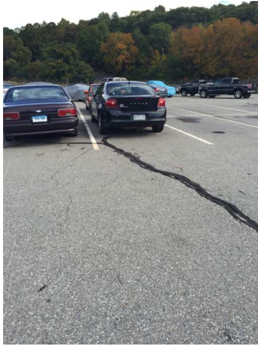
2A-1 Site 2A – Area A Landfill Deployed Parking Area Typical sealed and unsealed cracks
