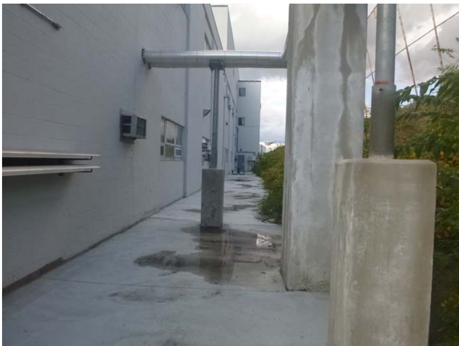
OU4-1 Lower Base – OU 4 Zone 7 Concrete cover placed behind Building 456.
