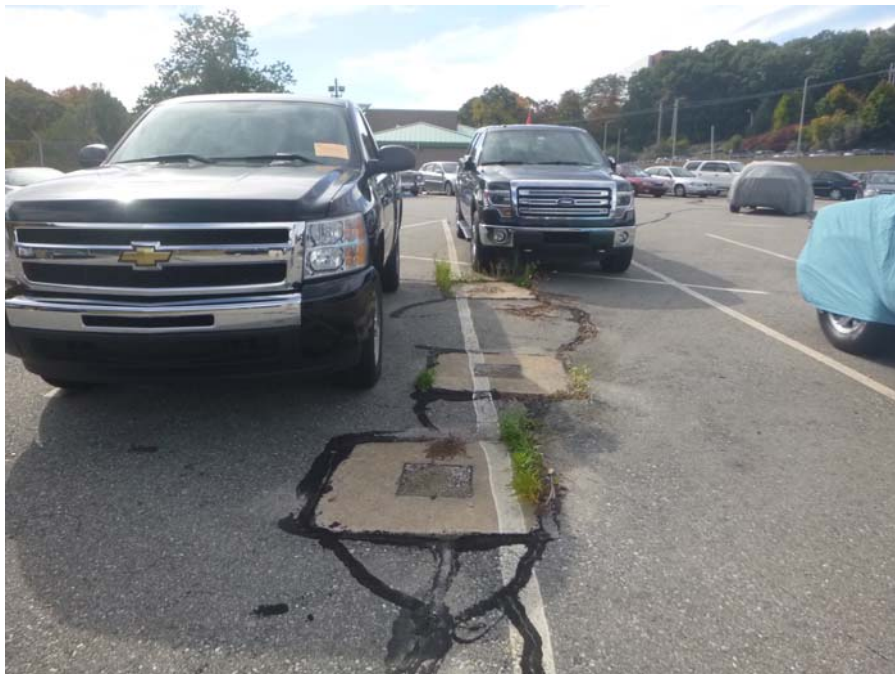
2A-2 Site 2A – Area A Landfill Deployed Parking Area Typical sealed and unsealed cracks, with vegetation
