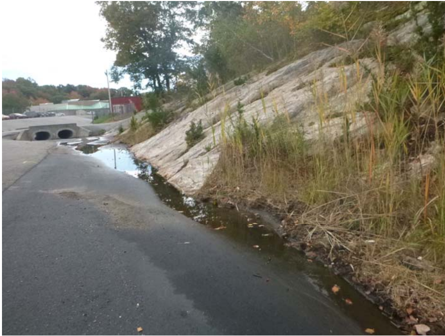
2A-15 Site 2A – Area A Landfill Drainage Channel A Drainage conditions indicating need for repaving
