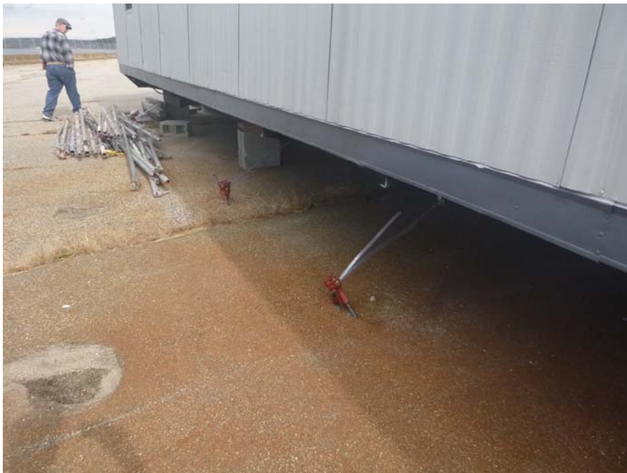
Site 6 – Former DRMO Cap Area Trailer tie-downs (rebar) potentially through cap
