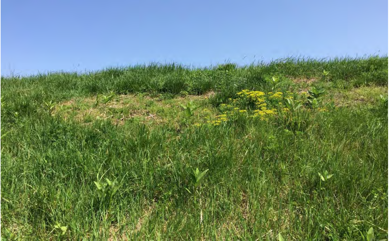
Photo #15: View of southern berm of Building 71 OPCA (photo direction North).
