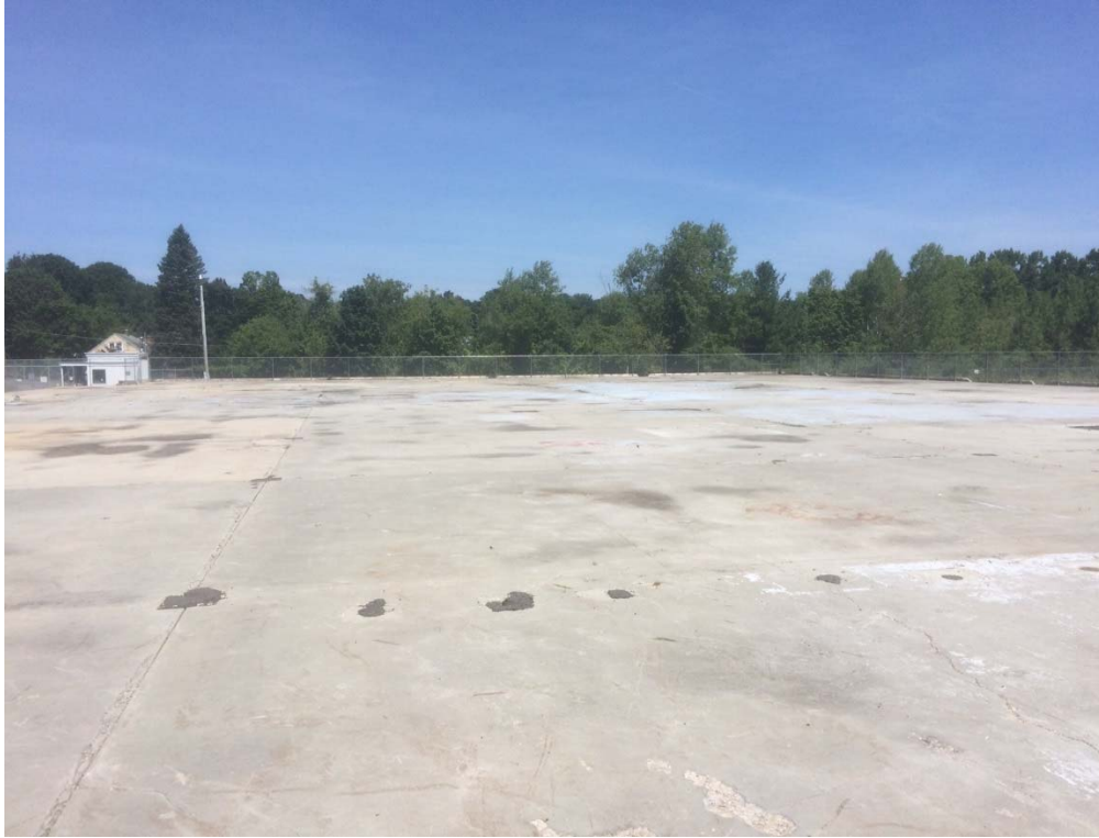
Photo #17: View of Building 9B Slab-Vegetation Removed.
