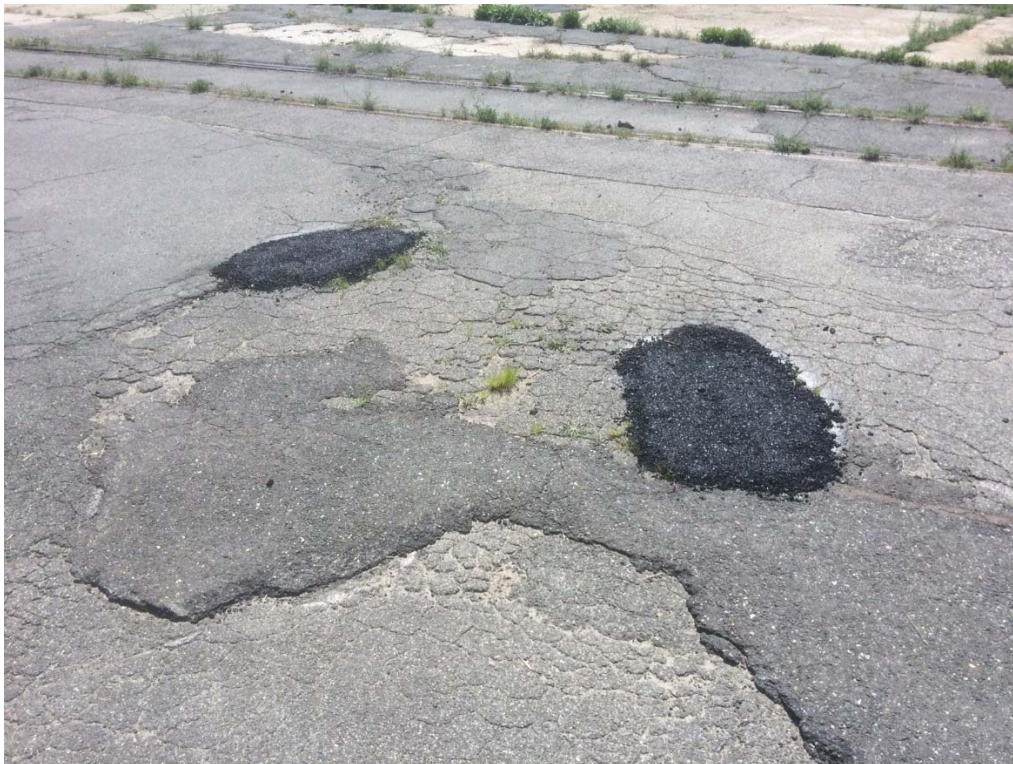
Photo #18: East Street Area 2 North Pavement Repair.
