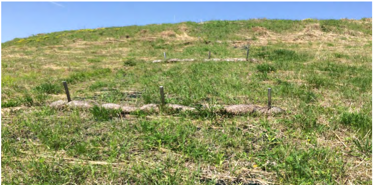
Photo #14: View of sediment and erosion control logs along southern edge of Building 71 OPCA (photo direction North).
