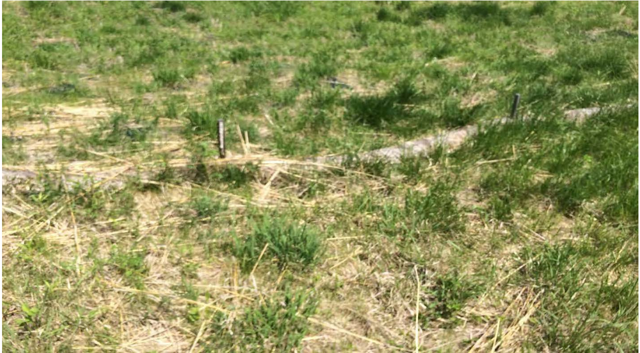
Photo #13: View of sediment and erosion control logs along southern edge of Building 71 OPCA (photo direction North).
