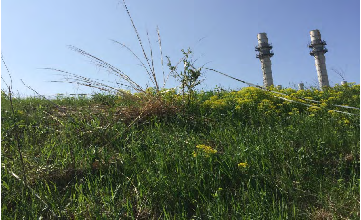
Photo #5: View of berm along the west side of the Building 71 OPCA (photo direction East).
