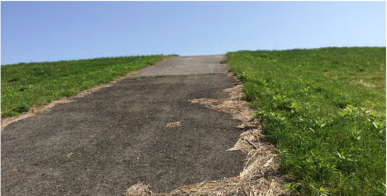
Photo #16: View of access road to top of Building 71 OPCA (photo direction North).
