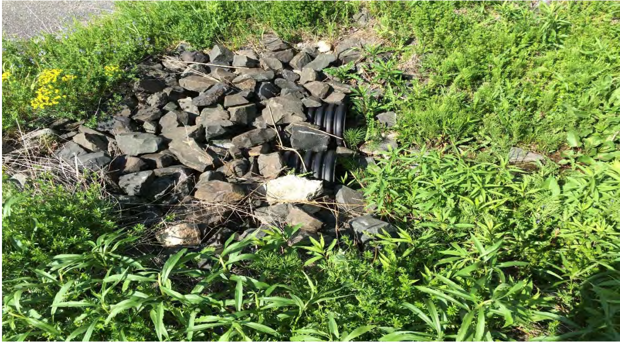
Photo #10: View of Anchor trench drain pipes in berm of Building 71 OPCA (photo direction North).
