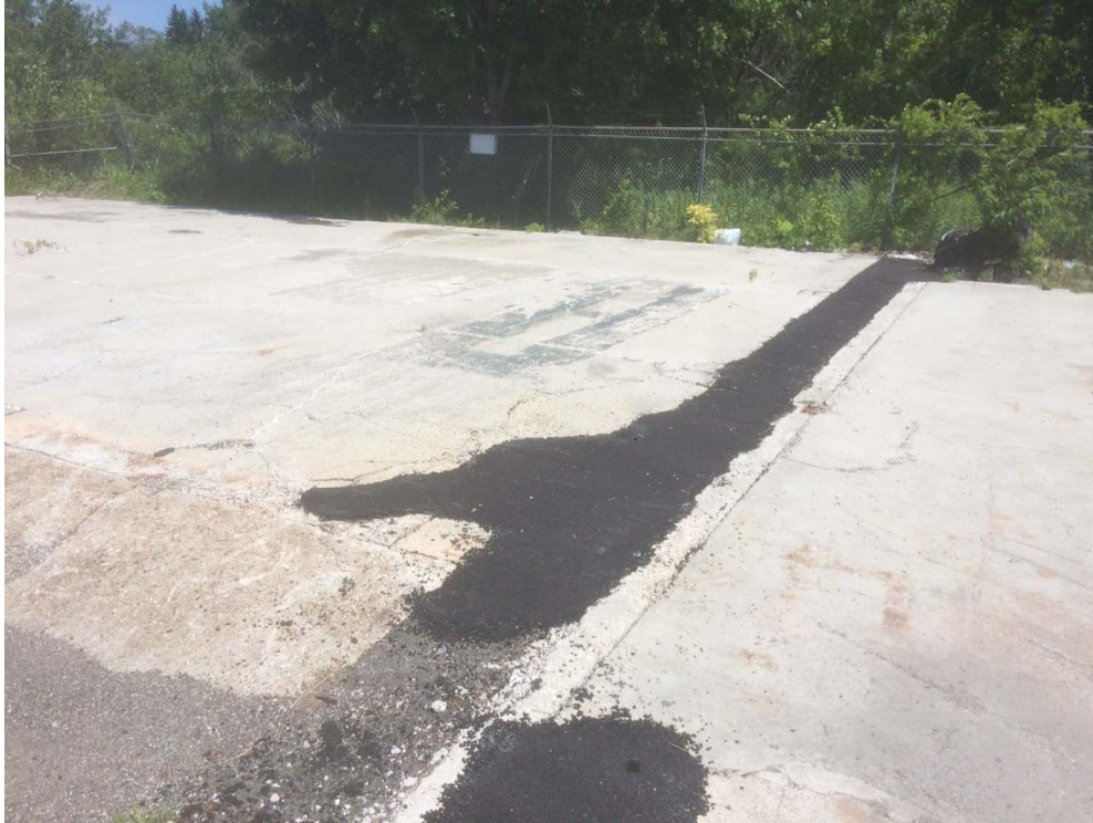
Photo #19: Pavement Repair Between Buildings 9B and 9F.
