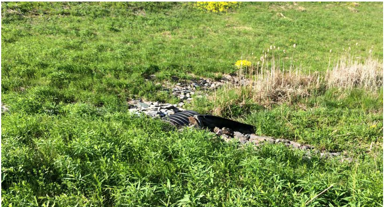
Photo #6: View of North Stormwater Basin drain pipes (photo direction West).
