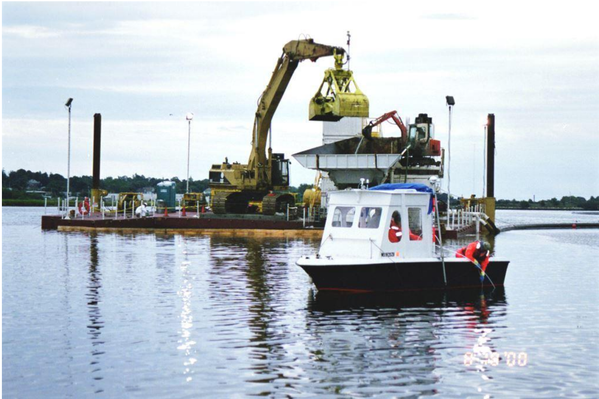
Hybrid Dredging Operation (similar to this) will be mobilized for 2017 in Upper Harbor
