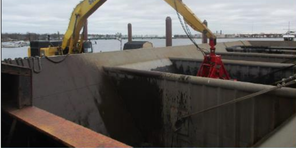
1 Mechanical dredging in area H36 within Cozy Cove.
