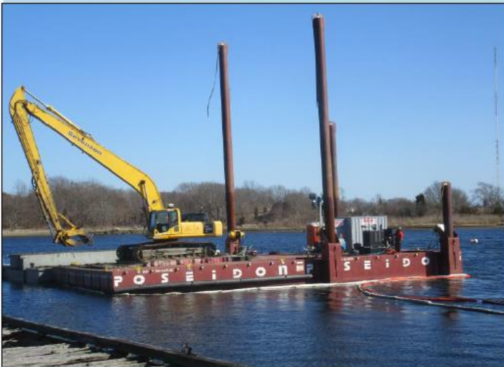
1 Mechanical dredging in area H36 within Cozy Cove.
