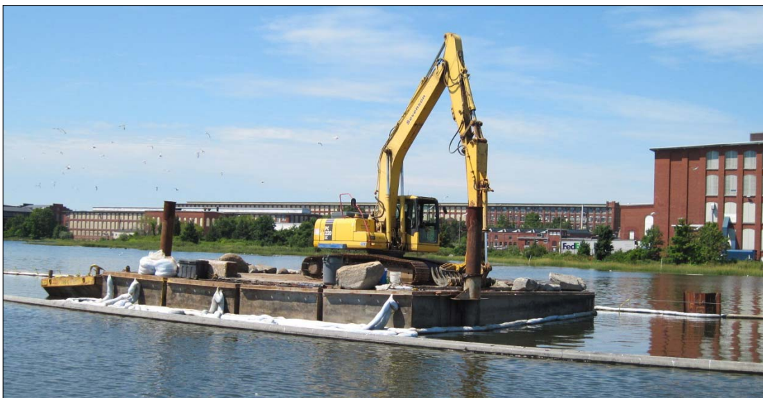
Figure 8. Debris removal excavator and debris storage scow
