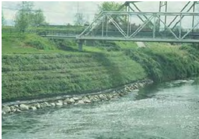
Photograph G-5. Vegetated geogrid with established vegetation.
