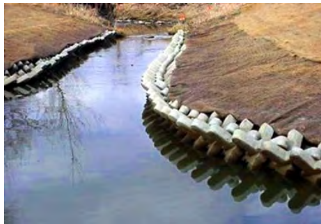
Photograph G-11. A-jacks along toe of bank.
