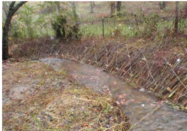
Photograph G-3. Newly installed brush mattress.
