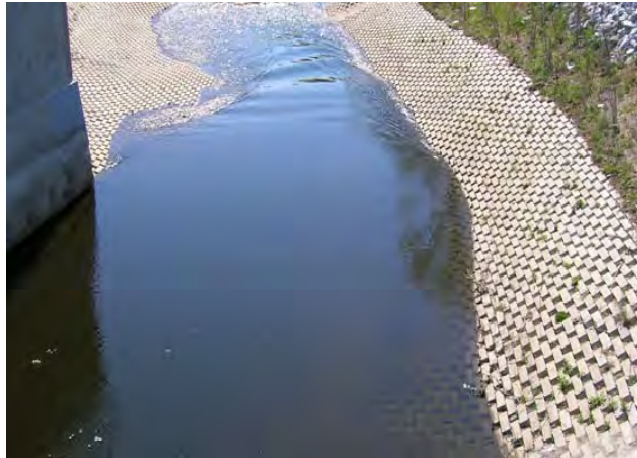
Photograph G-13. Articulated concrete block revetment on 1½ Mile Reach.
