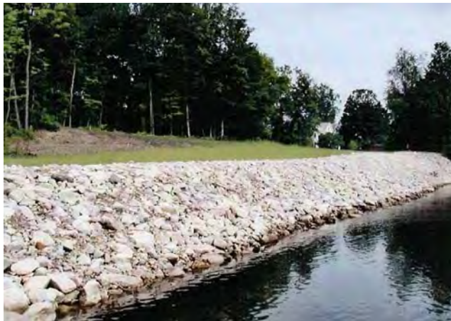
Photograph G-12. Riprap placed along entire bank.
