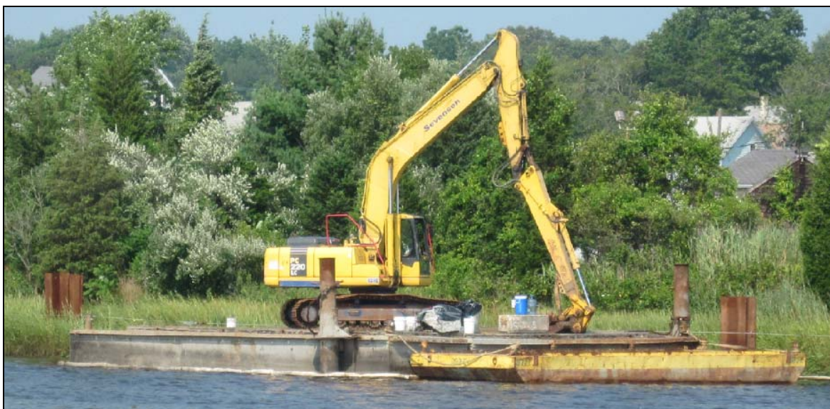
Figure 12. Debris removal excavator and debris storage scow
