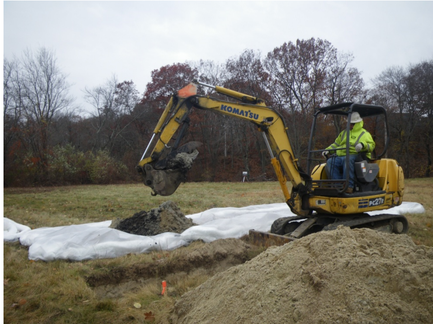
Figure B-3. Separation of Excavated Material from Above and Below the Geotextile Barrier
