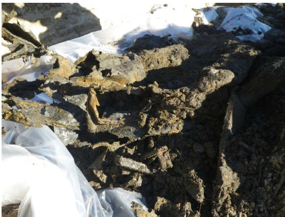
Figure B-7. Drum Carcasses from Test Pit at Transect 3, 85 – 95 Feet
