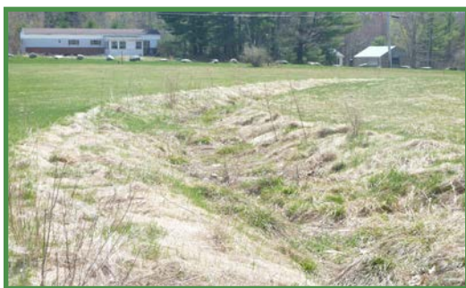
Figure 5: On-site drainage swale
