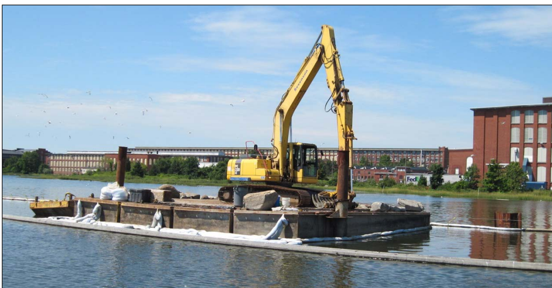
Figure 7. Debris Removal Excavator and Debris Storage Scow
