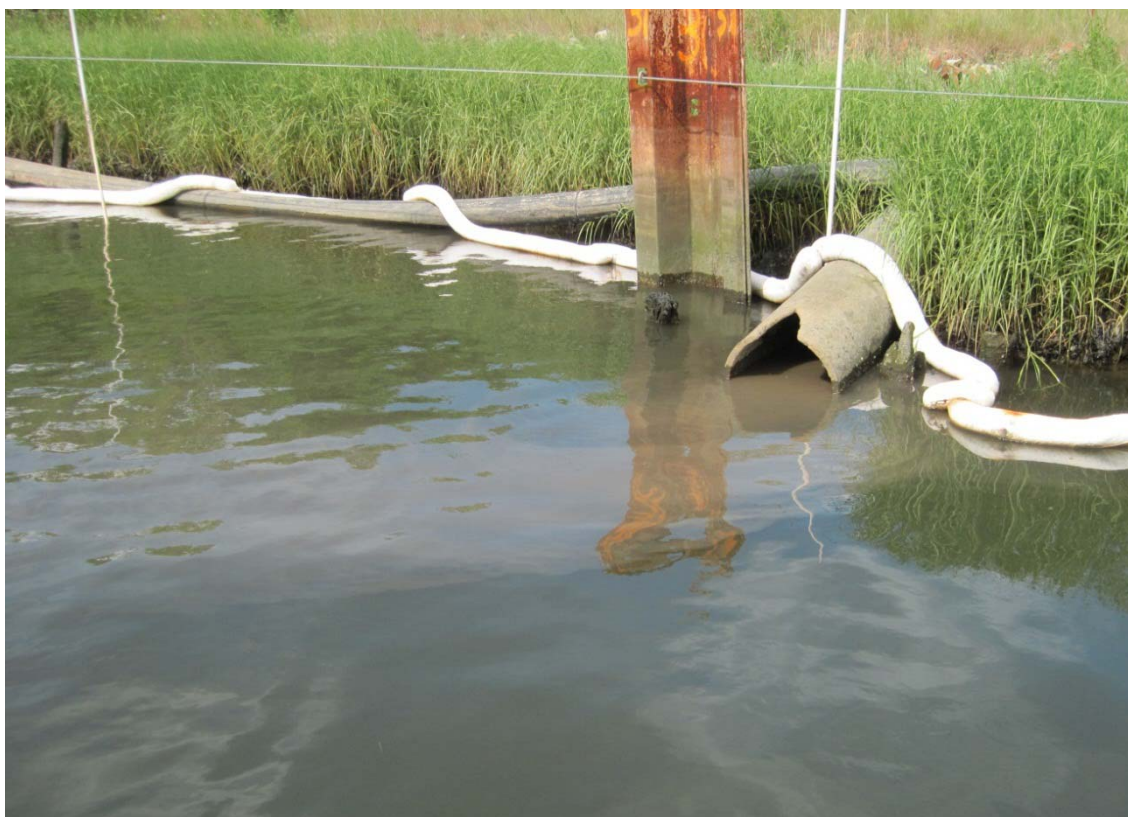
Figure 15. Sediment plume from drainage pipe caused by shore-based construction on 6/27.
