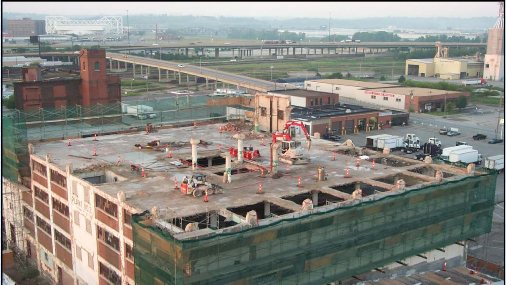
Demolition in Progress
