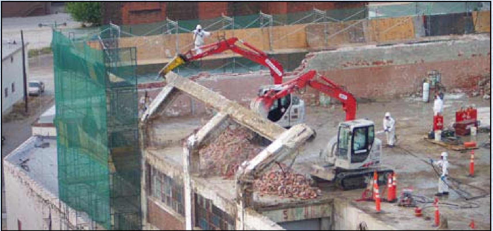
Demolition in Progress
