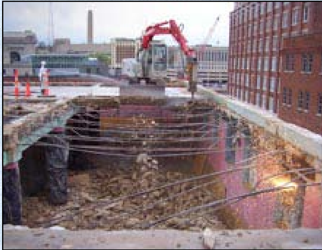
Demolition in Progress
