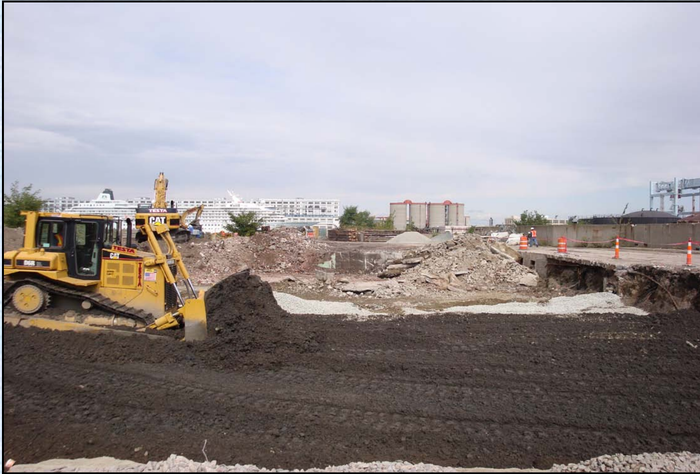
Placement of Fill
