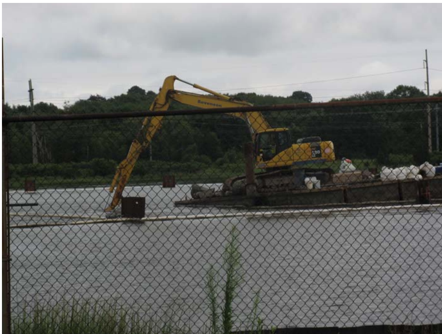
Photo 12: Mechanical Dredging to remove large debris from dredging area
