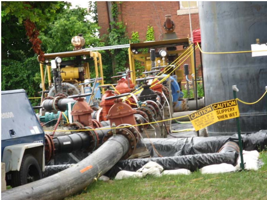
Photo 10: Desanding Operations
