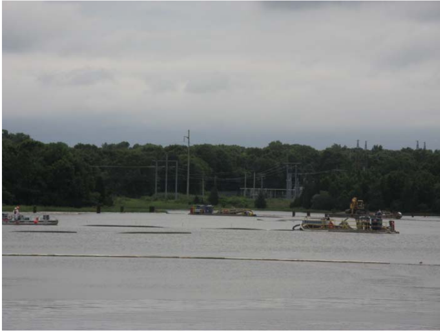
Photo 15: Wide view of dredging operations
