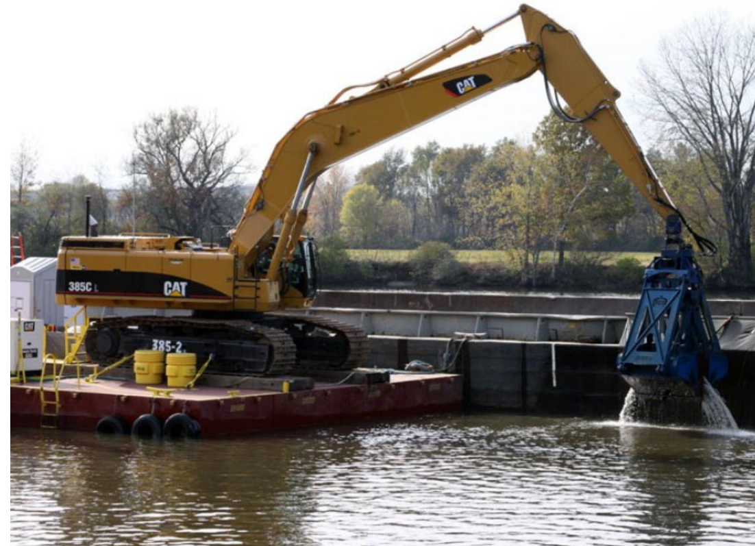
Dredging in the Hudson River ( image source )
