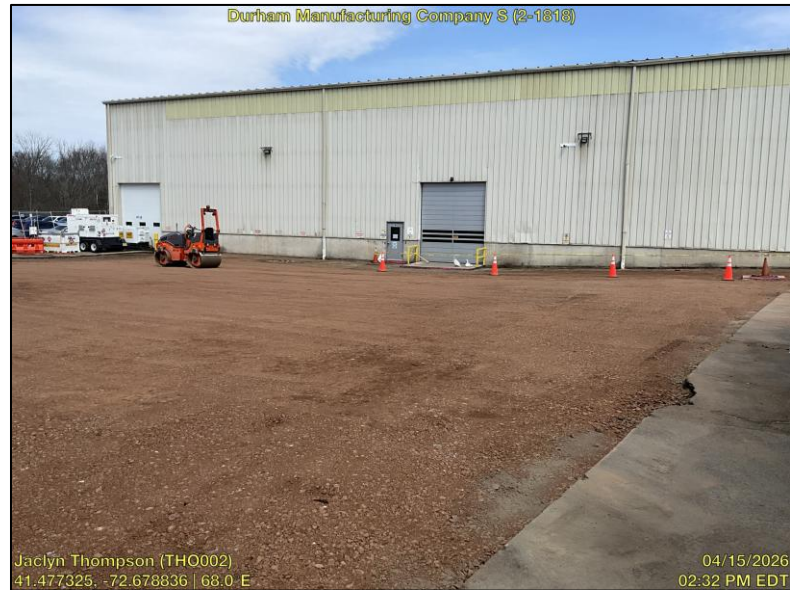
4/15: Preparation for binder installation in Phase 01B for temporary parking
