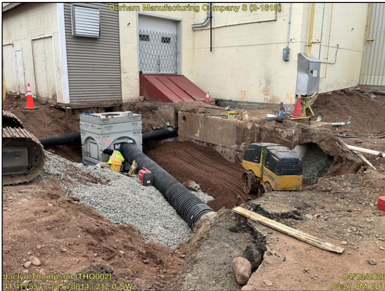
4/13: Restoration of utilities in Phase 01B
