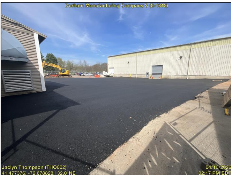
4/16: Placement of binder course on Phase 01B for temporary parking
