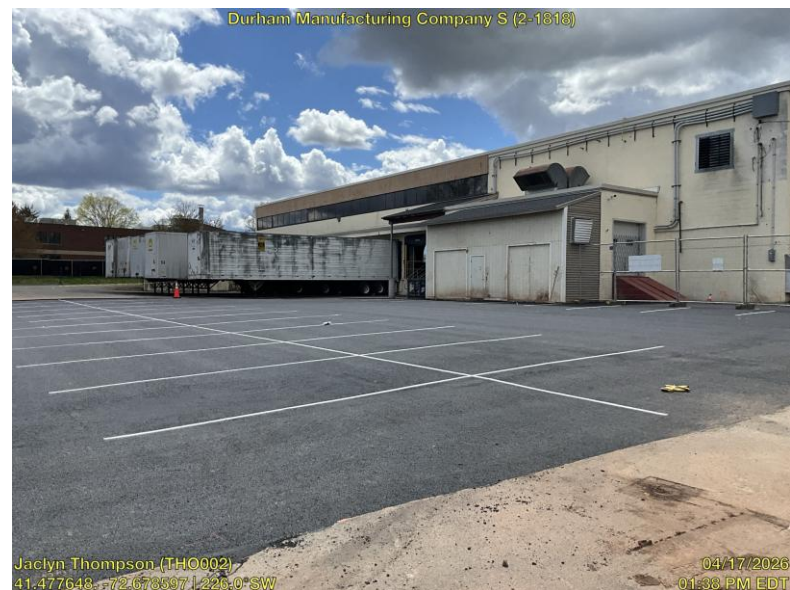
4/17: Placement of temporary parking lines in Phase 01B
