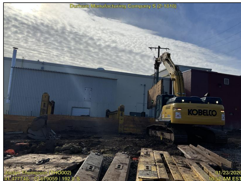
1/23: Relocation and installation of temporary trench support system along facility building
