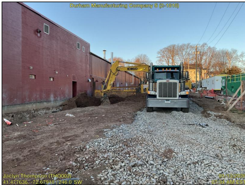
1/13: Excavation and exportation of Non-Hazardous material from Phase 01A
