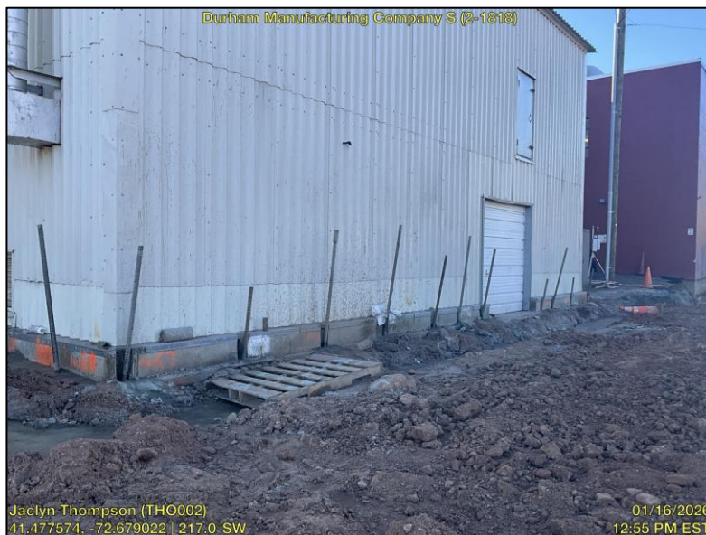
1/16: Installation of underpinning system along facility building
