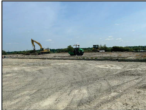
SCENE: Heavy equipment constructing a portion of the Pilot CDF cap.
