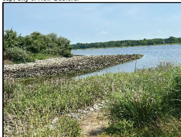
SCENE: Armor stone covering the Pilot Confined Disposal Facility (CDF) sediment cap, City of New Bedford.
