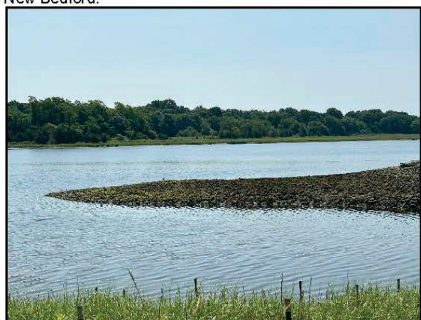
SCENE: Armor stone covering the "Crib Cap" sediment cap, City of New Bedford.
