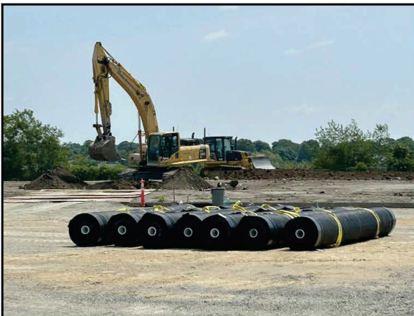
SCENE: Staging area for geotextile liners to be installed as part of the Pilot CDF cap.
