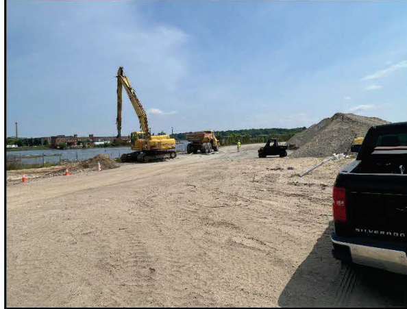
SCENE: Heavy equipment excavating fill material used for shaping and grading the Pilot CDF cap.
