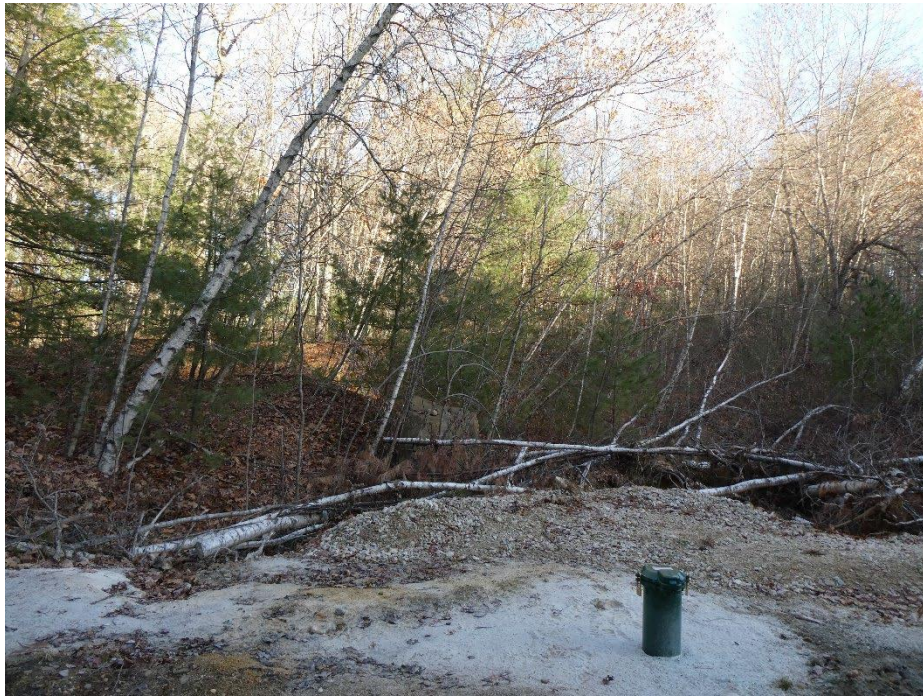
New bedrock monitoring well for current investigations
