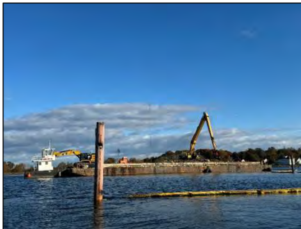
Dredging at CAD Cell #4.
