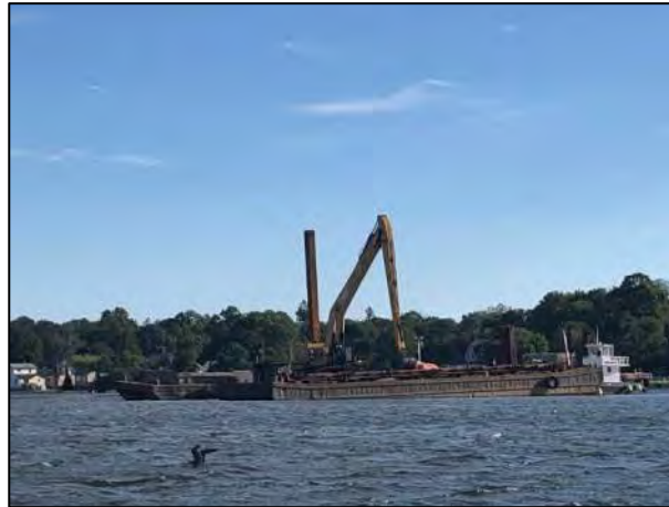
Dredging at CAD Cell #4.
