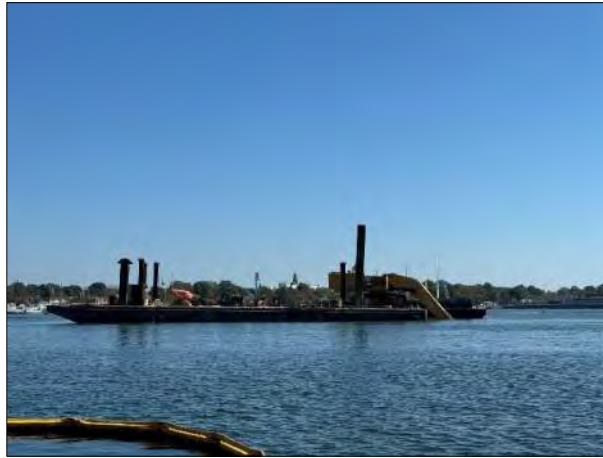
Dredging at CAD Cell #4.
