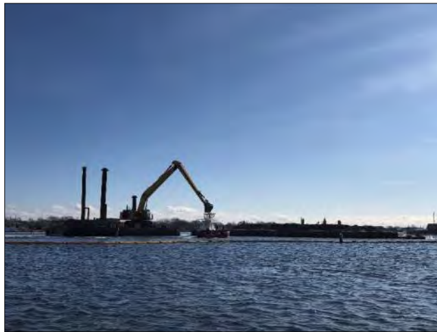
Dredge PC-1250 dredging at CAD Cell #4.
