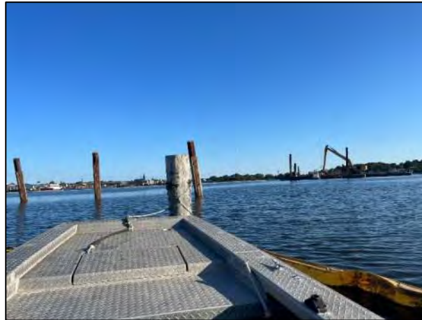
Bed Leveling at LHC.
