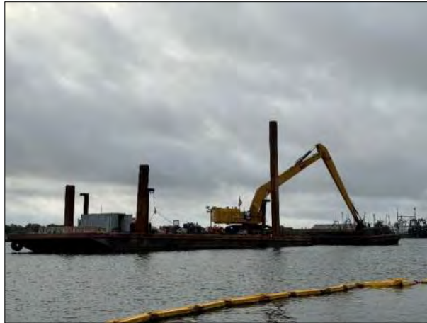
Dredging at CAD Cell #4.
