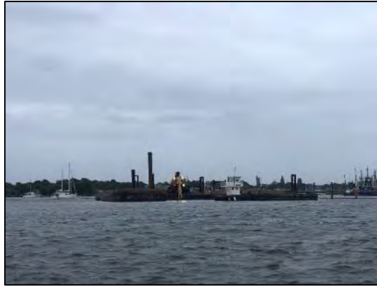
Dredging at CAD Cell #4.
