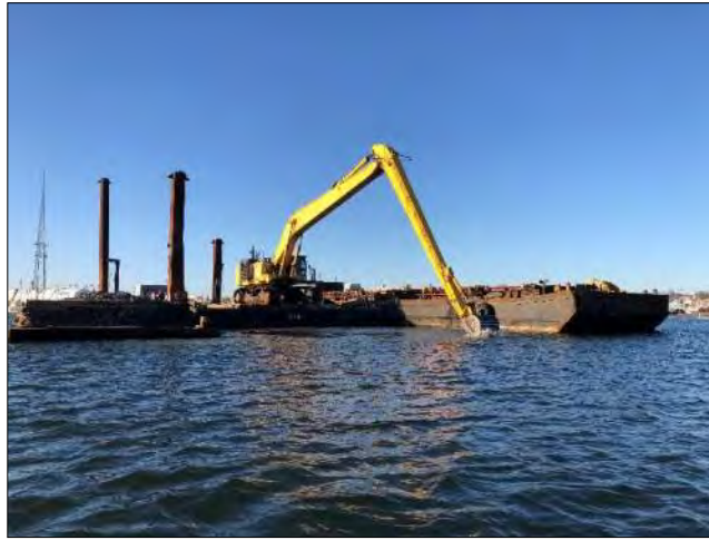
Dredge PC-1250 dredging at CAD Cell #4.
