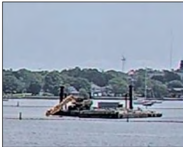
Dredge PC-1250 dredging at CAD Cell #4.
