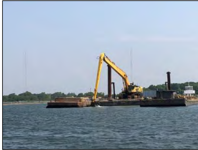
Dredge PC-1250 dredging at CAD Cell #4.
