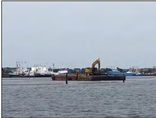
Bed Leveling at LHC.
