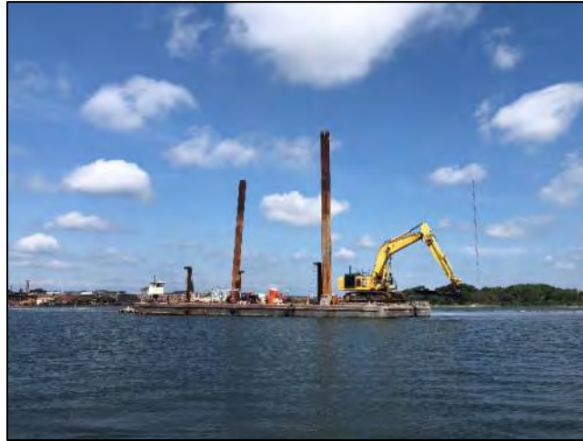
Dredge PC-1250 Bed Leveling at LHCC.
