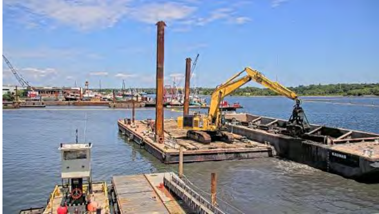
Dredge PC-1250 at North Terminal Pre-Cell Dredge Area
