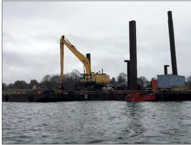
Dredge PC-1250 dredging at CAD Cell #4.
