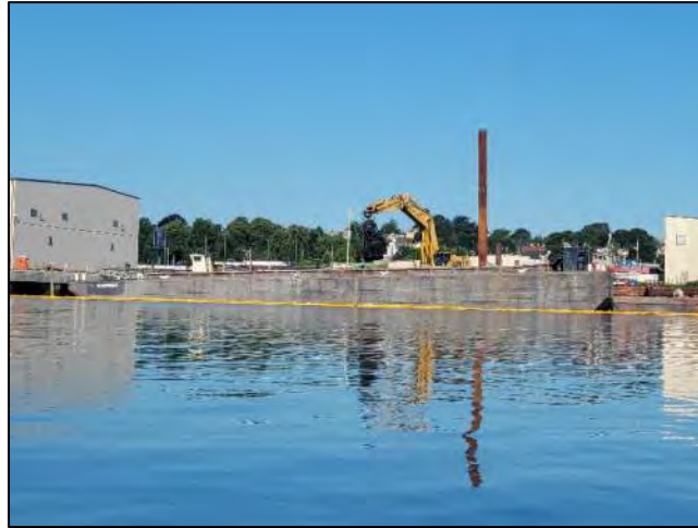
Dredge PC-1250 at North Terminal Pre-Cell Dredge Area
