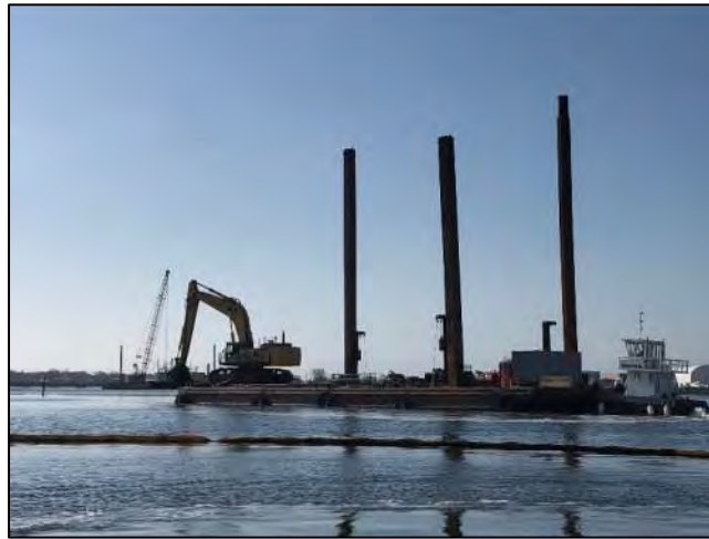
Dredge PC-1250 bed leveling at LHCC.
