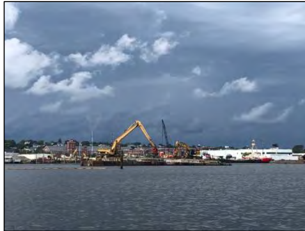
Dredging at CAD Cell #4.
