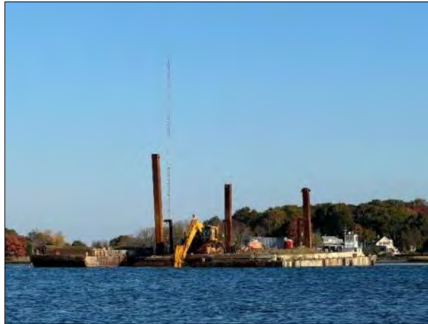
Dredging at CAD Cell #4.
