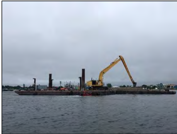
Dredge PC-1250 dredging at CAD Cell #4.
