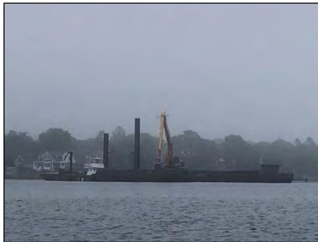
Dredge PC-1250 dredging at CAD Cell #4.
