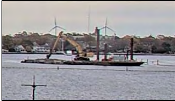
Dredging at CAD Cell #4.
