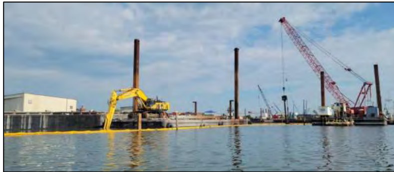
Dredge PC-1250 at North Terminal Pre-Cell Dredge Area
