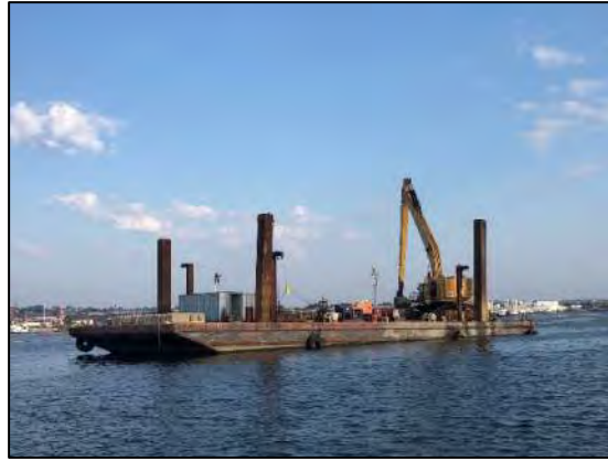
Dredging at CAD Cell #4.
