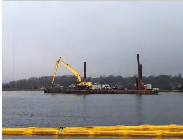
Dredge PC-1250 dredging at CAD Cell #4.
