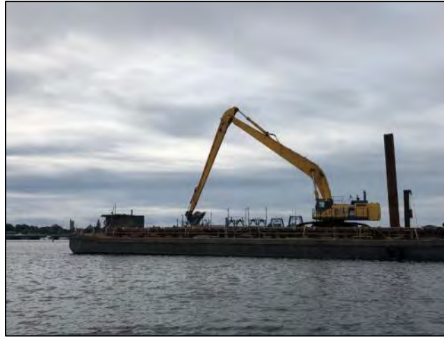
Dredge PC-1250 dredging at CAD Cell #4.
