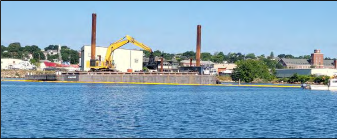
Dredge PC-1250 at North Terminal Pre-Cell Dredge Area
