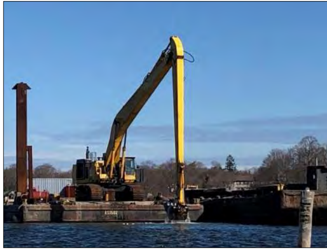
Dredge PC-1250 dredging at CAD Cell #4.
