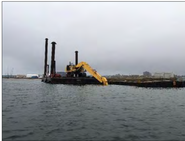
Dredge PC-1250 dredging at CAD Cell #4.
