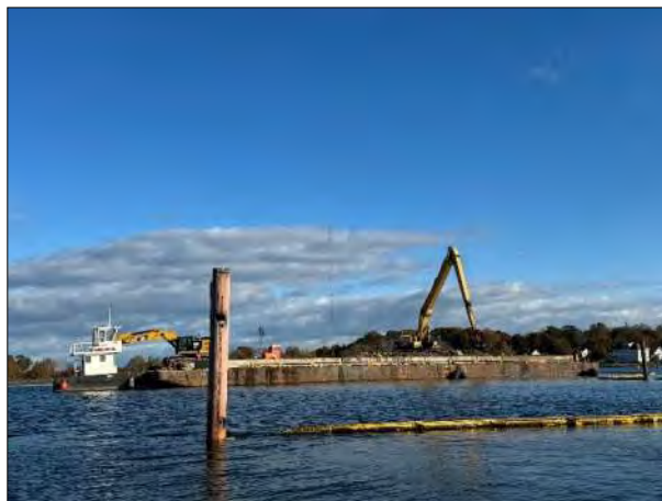
Dredging at CAD Cell #4.
