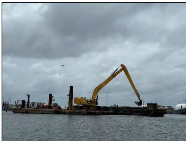
Dredging at CAD Cell #4..
