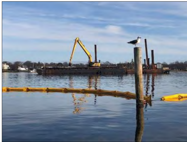
Dredge PC-1250 dredging at CAD Cell #4.
