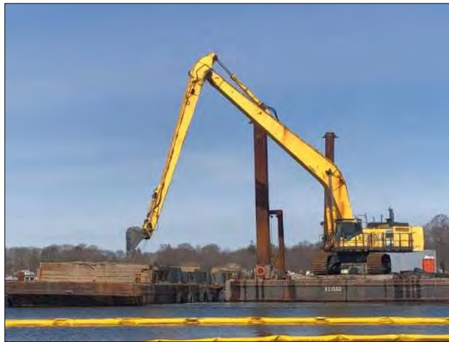
Dredge PC-1250 dredging at CAD Cell #4.
