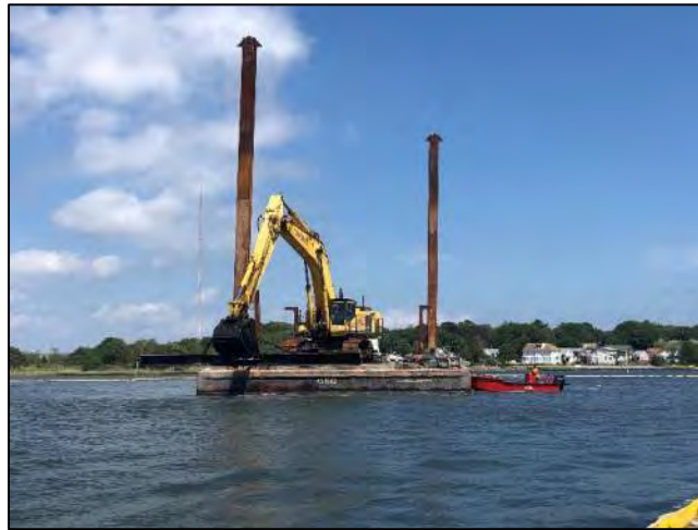
Dredge PC-1250 Bed Leveling at LHCC.
