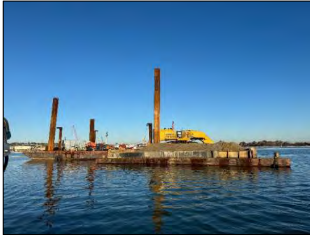
Dredging at CAD Cell #4.
