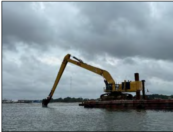
Dredging at CAD Cell #4.
