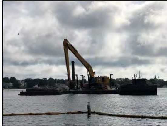
Dredging at CAD Cell #4.
