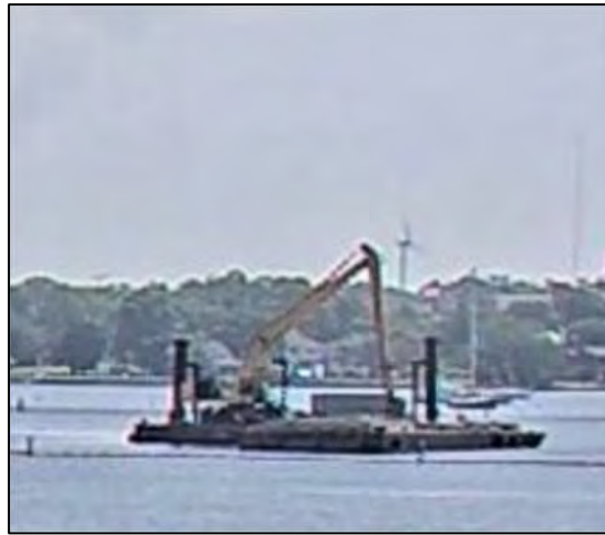
Dredge PC-1250 dredging at CAD Cell #4.
