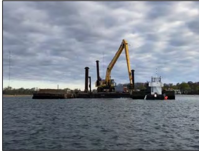
Dredge PC-1250 dredging at CAD Cell #4.
