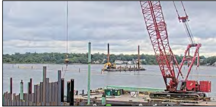
Dredge PC-1250 Bed Leveling at LHCC.
