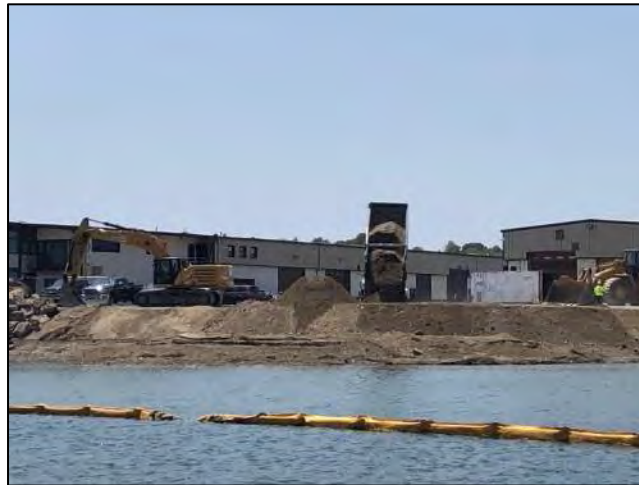
Dredge PC-1250 dredging at CAD Cell #4.
