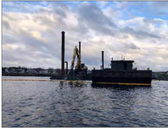
Dredge PC-1250 dredging at CAD Cell #4.
