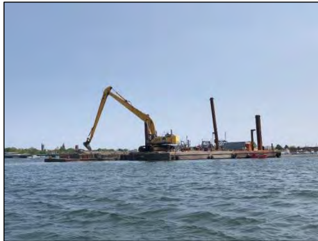
Dredge PC-1250 dredging at CAD Cell #4.
