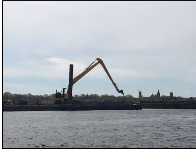
Dredge PC-1250 dredging at CAD Cell #4.
