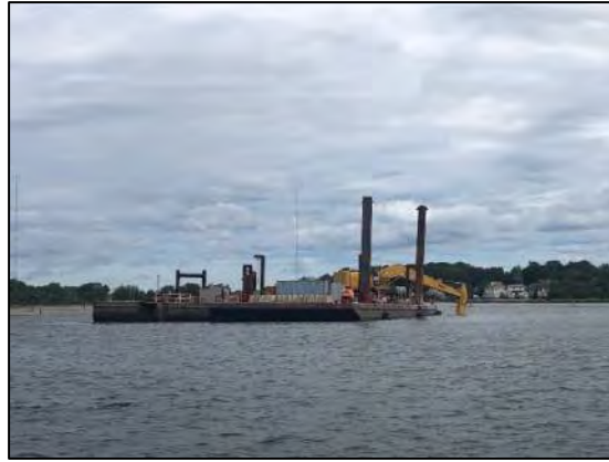
Dredging at CAD Cell #4.
