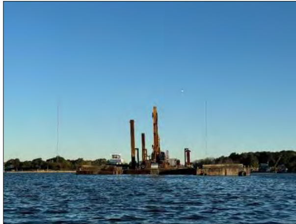
Dredging at CAD Cell #4.
