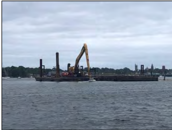
Dredging at CAD Cell #4.
