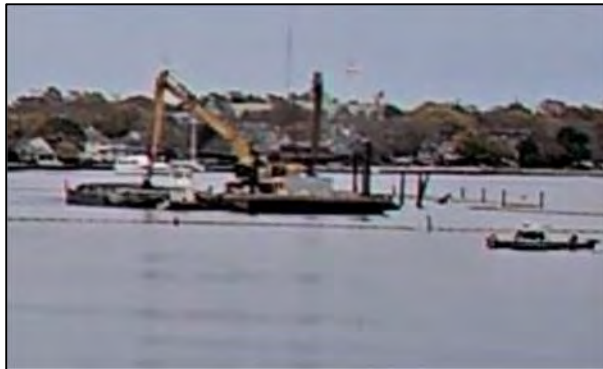
Dredging at CAD Cell #4.
