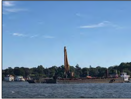
Dredging at CAD Cell #4.
