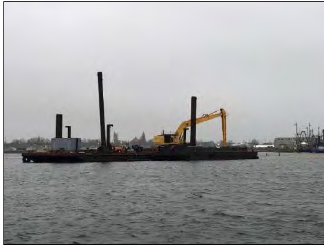
Dredge PC-1250 dredging at CAD Cell #4.
