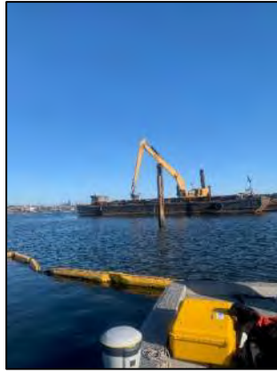
Dredging at CAD Cell #4.
