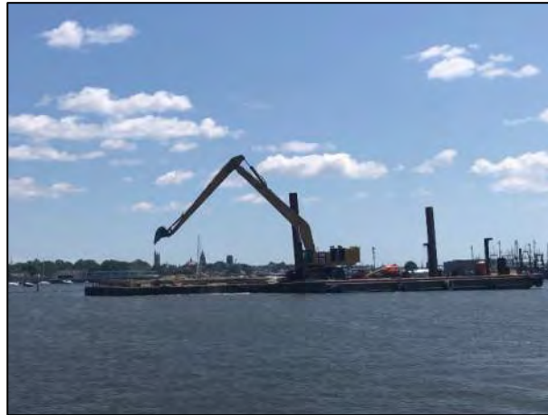
Dredging at CAD Cell #4.
