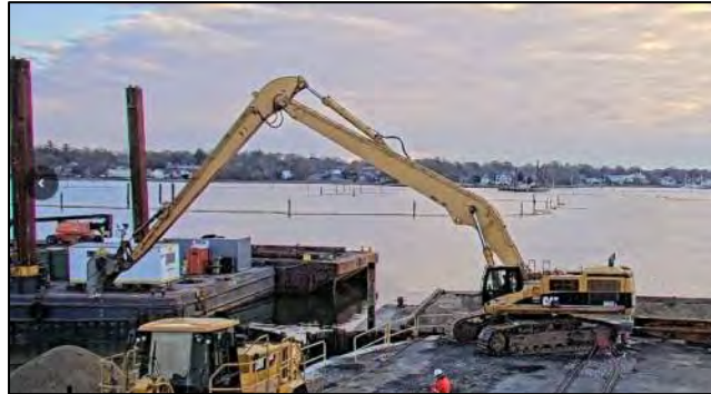
Landside excavator loading deck barge dredged material into cofferdam cell #1.
