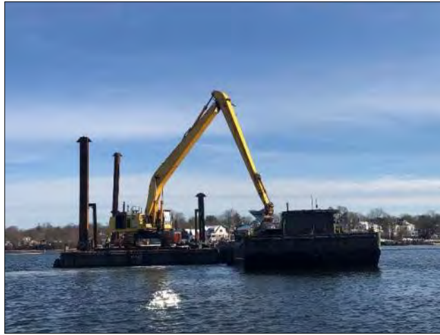
Dredge PC-1250 dredging at CAD Cell #4.
