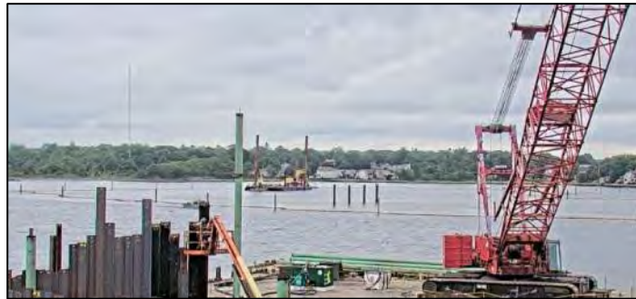
Dredge PC-1250 Bed Leveling at LHCC.
