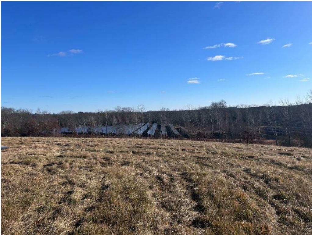
Landfill cap with the solar facility in background
