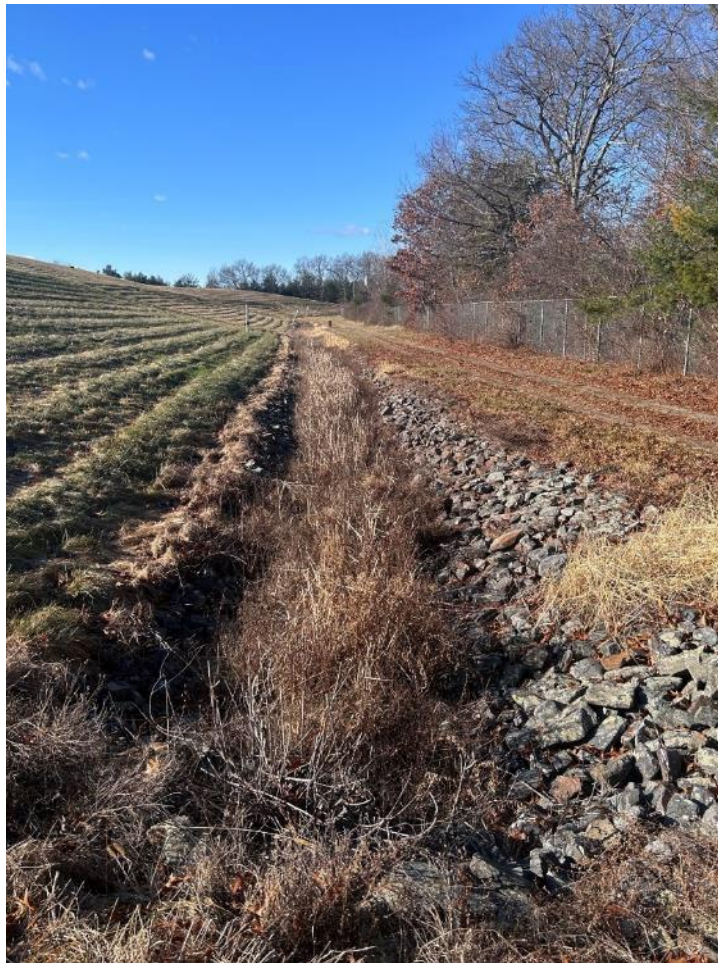
Stormwater drainage with some vegetative growth
