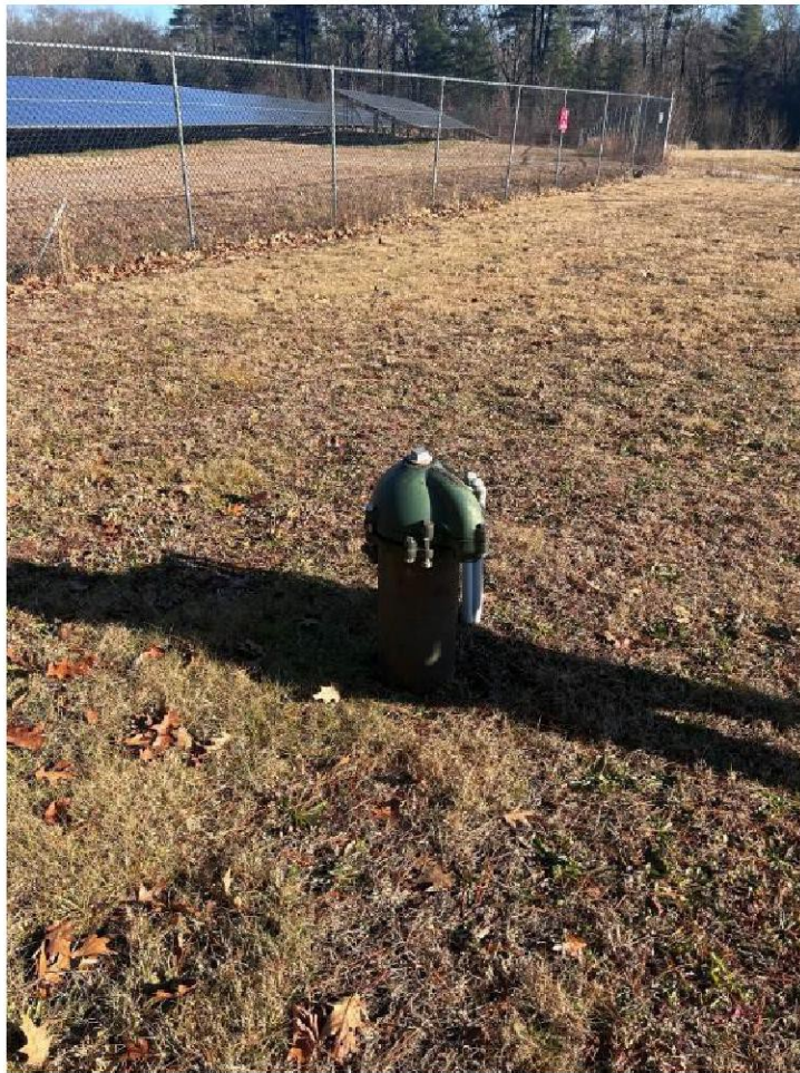
Inactive pumping well on Concord Bus Facility
