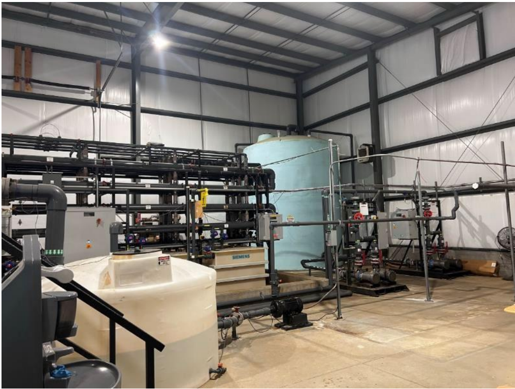
Interior of the LATS building
