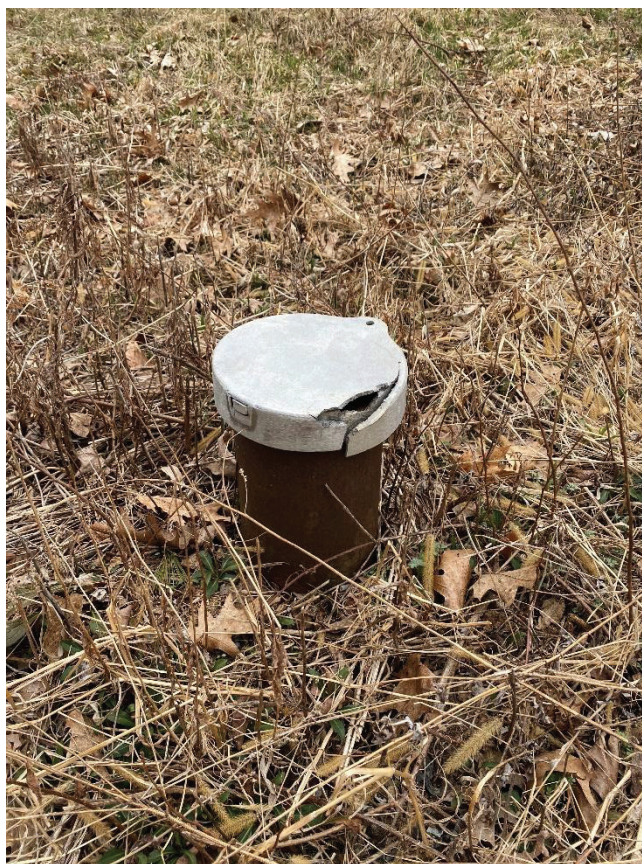
Damaged well lid in the MW-101 well cluster
