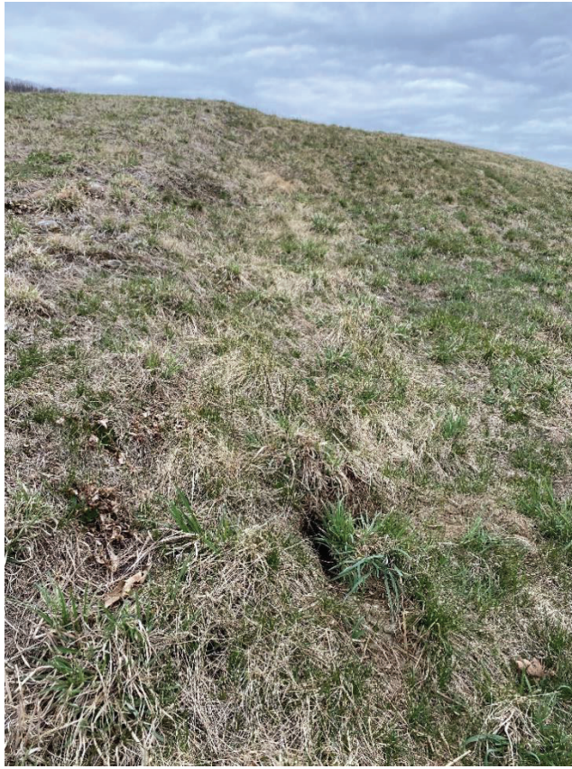
Small animal burrow on the southern slope of the landfill
