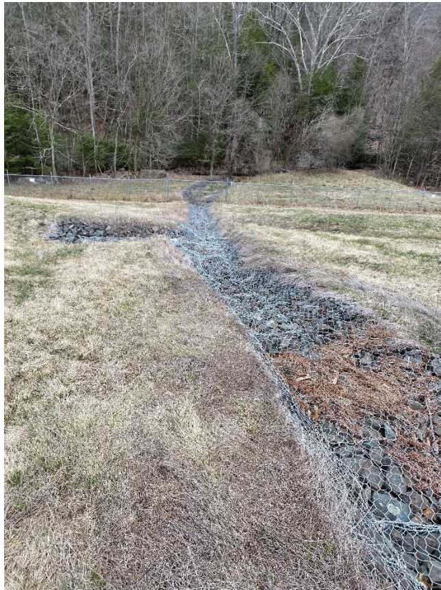
Riprap drainage channel on the western slope of the landfill
