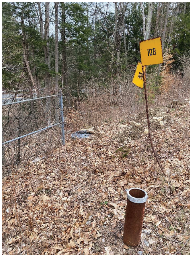
Well MW-108 missing a well cap
