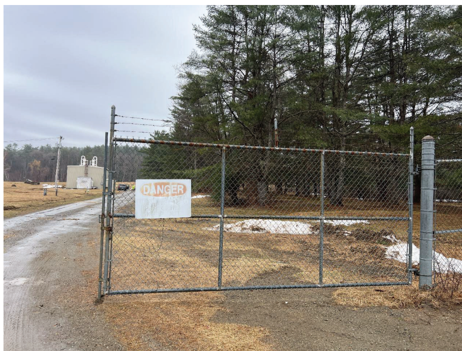
Second entrance to landfill property
