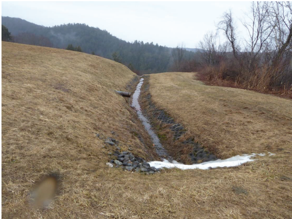
Downchute after the sedimentation pond
