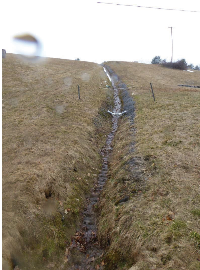
Central downchute where recent erosion work was completed
