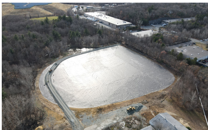
Aerial image of the Containment Area feature (engineered slurry wall and temporary cap) on the Olin property facing south, December 2021. The PRPs replaced the previous cover of the Containment Area in the fall of 2021.
