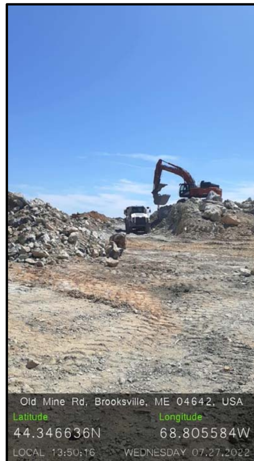
Photo 1 (group). Excavating, hauling, and downsizing oversized rock at WRP#3.
