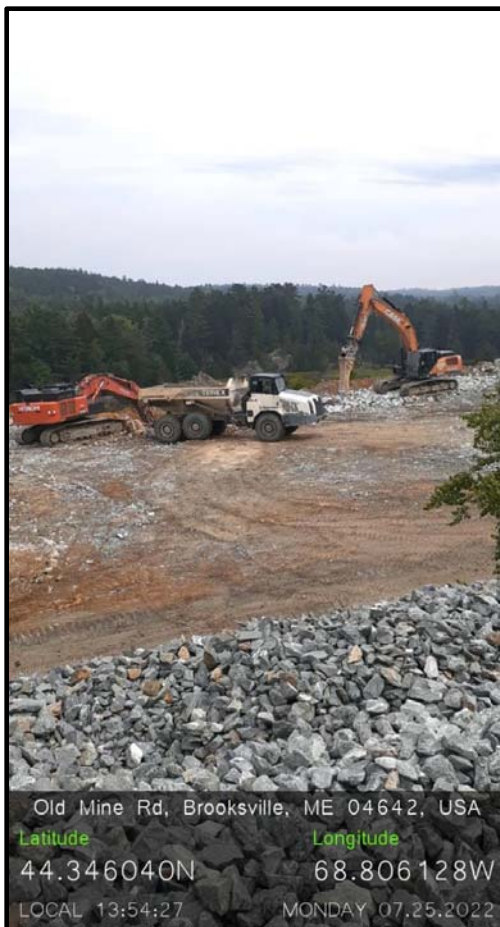
Photo 1 (group). Excavating, hauling, and downsizing oversized rock at WRP#3.
