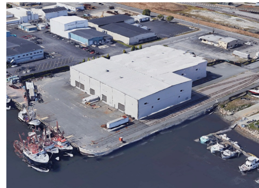
After the contaminated sediments were dried out in the dewatering facility, they were transported by rail to a secure landfill in Michigan (image from Google Maps)
