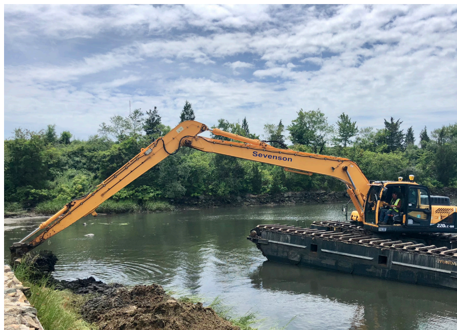
Excavation of contaminated shoreline, Fairhaven, Massachusetts (courtesy of Sevenson Environmental Services)
