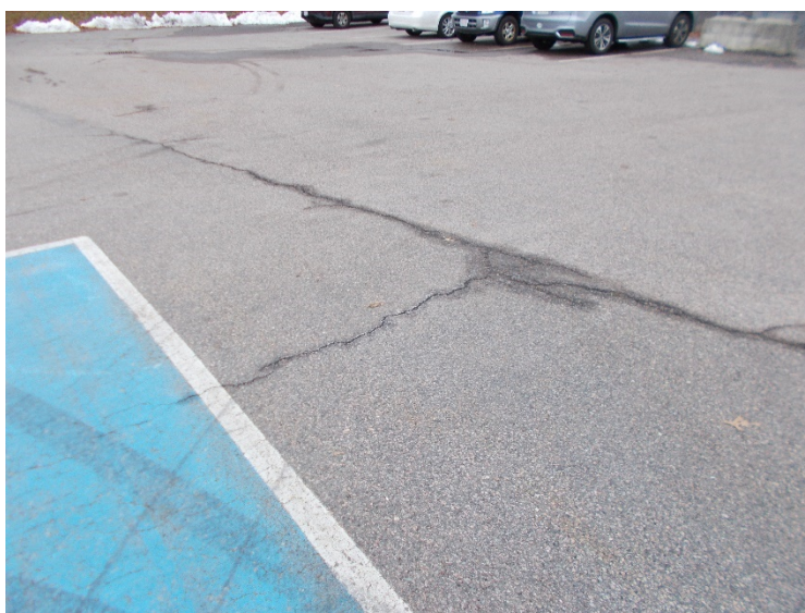
Photo #2: Cracks in pavement in Asphalt cover, Foxborough/ Parking Lot
