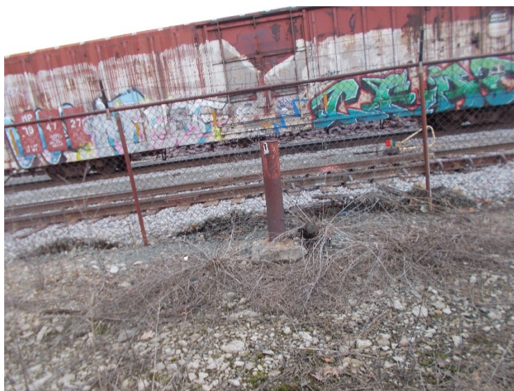
Photo #14: Monitoring Well along Railroad fencing; Well in good condition and secured.
