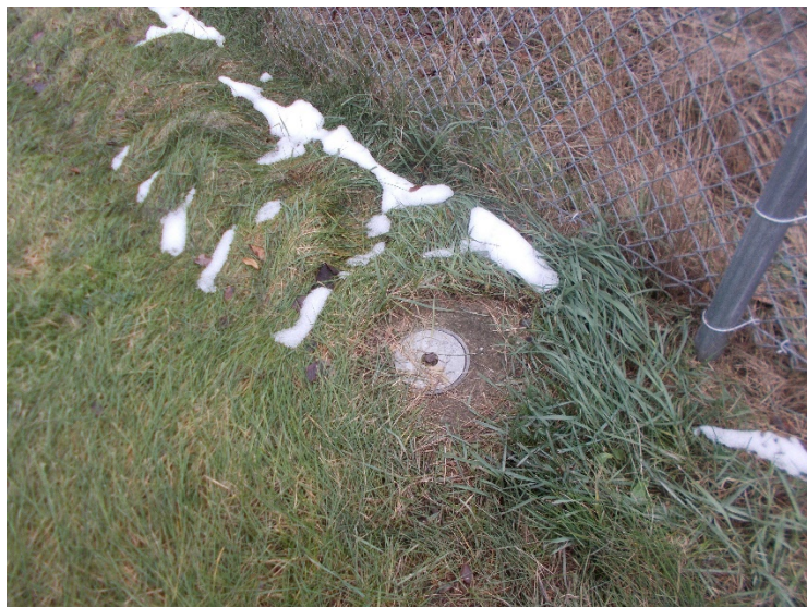
Photo #13: Monitoring Well on Northeast quadrant of Mansfield portions of the Site; well secured and in good condition.
