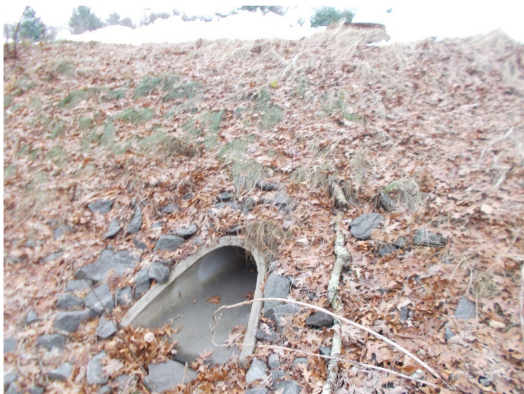
Photo #3: Stormwater control structure on Foxborough property. Drainage area clear; no obstructions noted.
