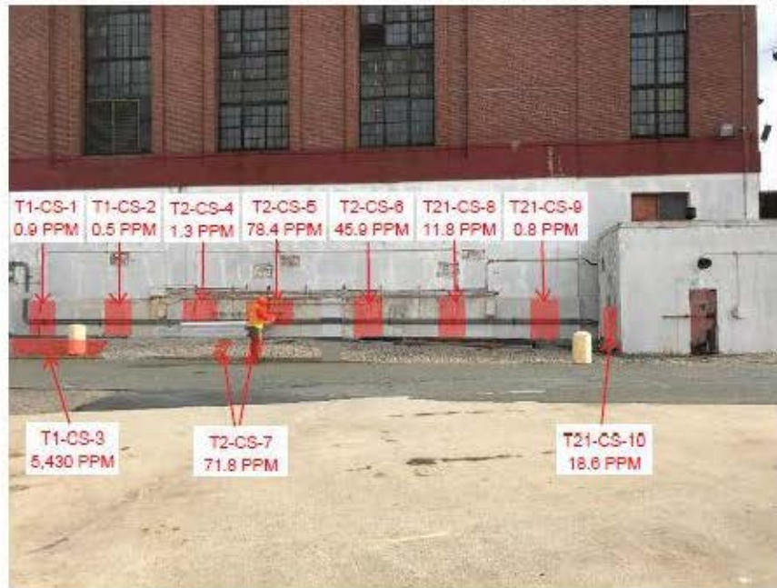
Photo 1- Transformer 1, 2, and 21 Area looking north at Mystic 1 building
