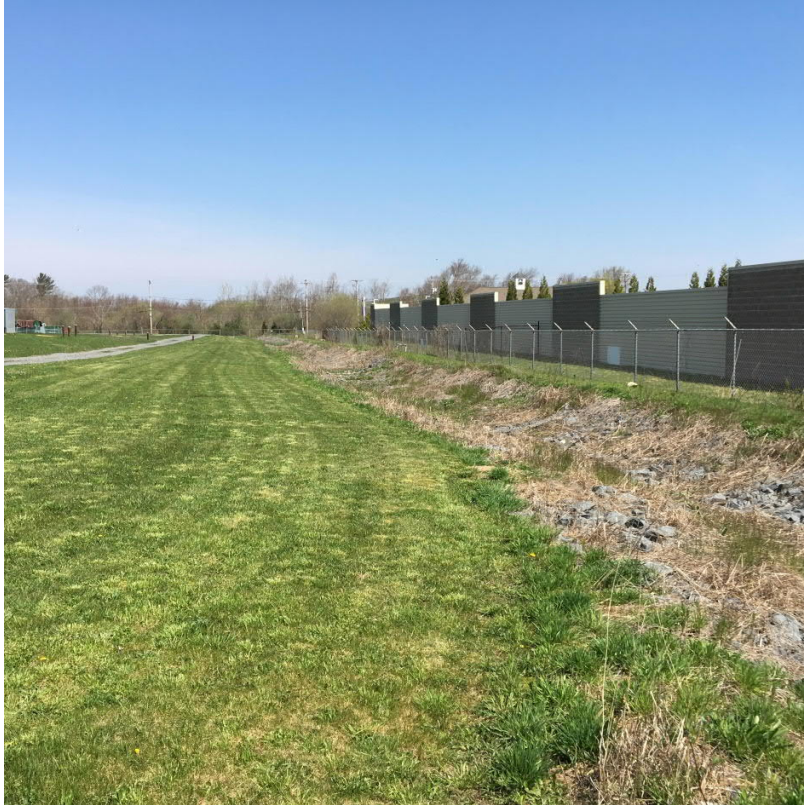
Rip-rap lined eastern cap swale is in good condition
