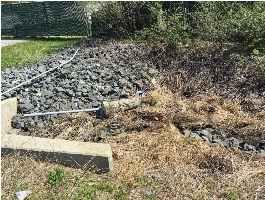
Inlet #3 in northeast corner of site receives run-on from off-site to the east. Note iron floc in wet area in center of photo.
