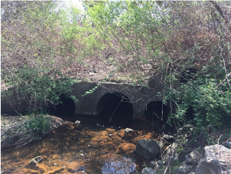
View of headwall on north side of Hathaway Road.
