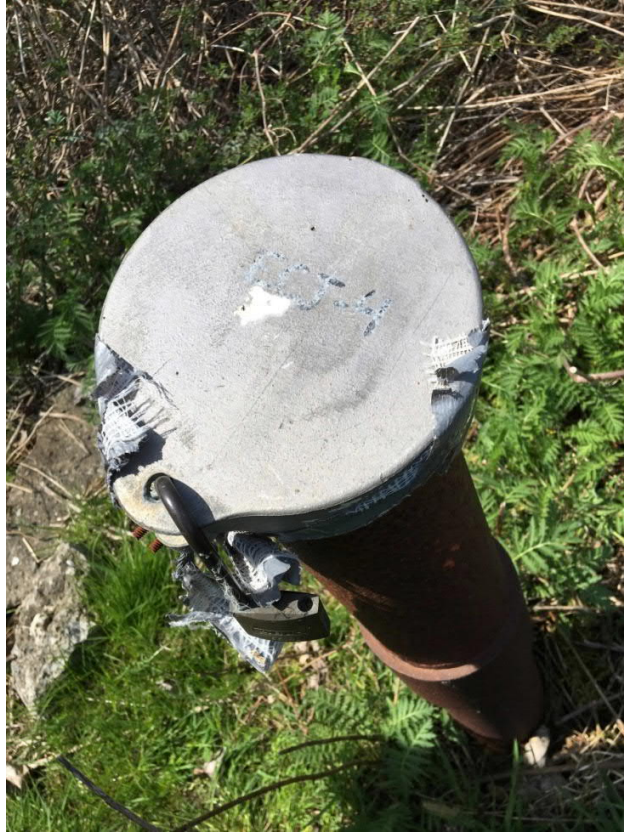
Well ECJ-4, located in golf course, not locked.
