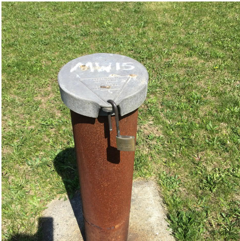
Monitoring well MW-15 is not locked.
