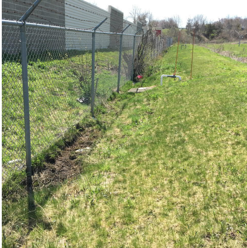
View of eastern fence line looking south and gas monitoring well GM-19.
