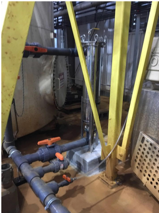
Bag filter in center of photo was installed by the City in December 2017 to provide additional solids removal at the end of the treatment process.
