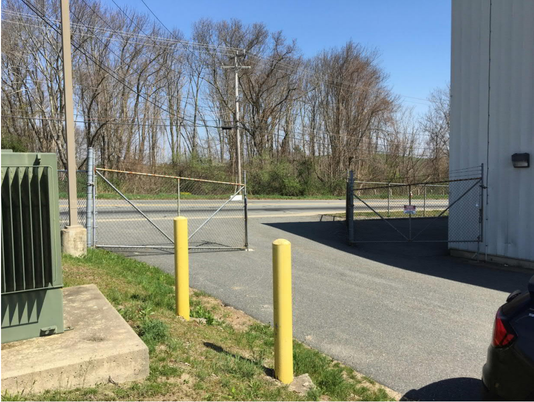
Swing gates at GWTP entrance are in adequate condition.
