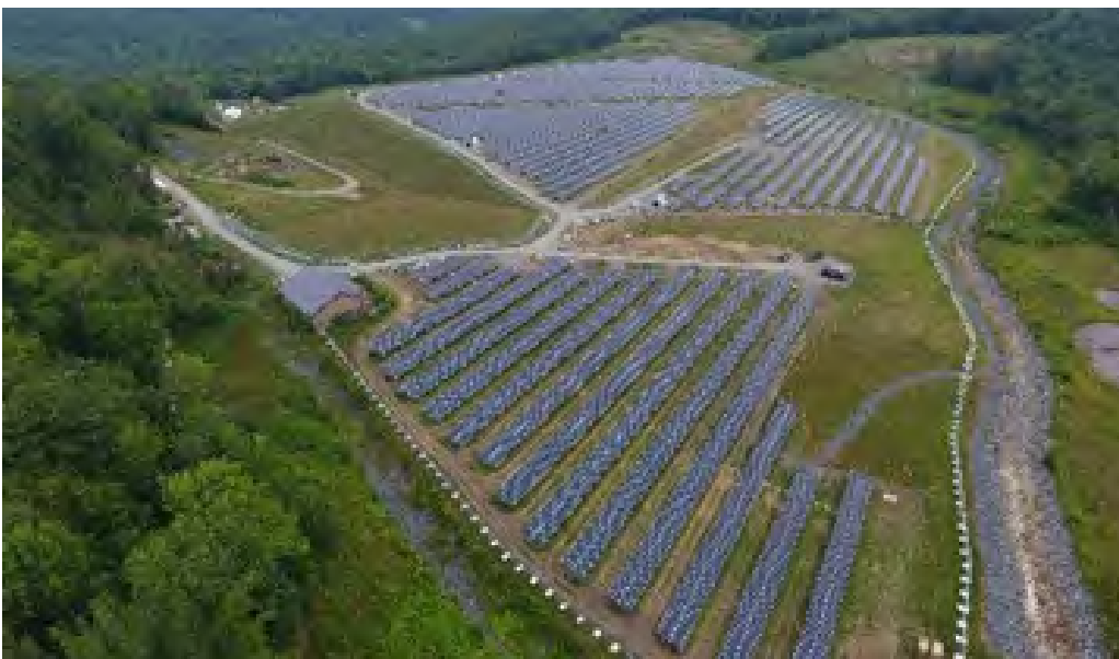
Figure 18. Aerial view of the solar array at the Elizabeth Mine site (Vermont). Image used with permission of Weston and Sampson, Conti Solar, and Elizabeth Mine Solar I, LLC.
