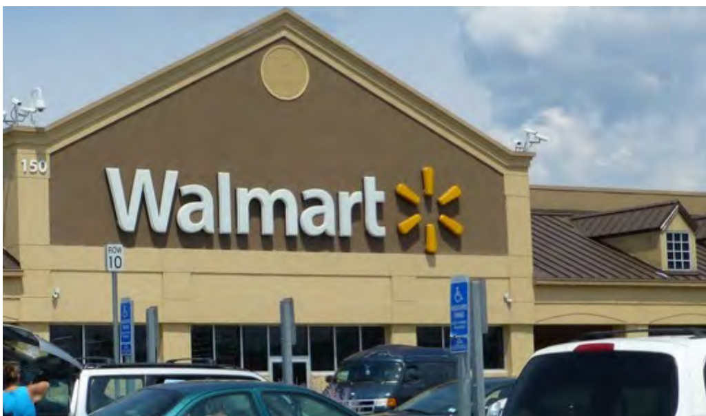
Figure 24. The Walmart store at the Stratford Crossing Shopping Center (Connecticut).
