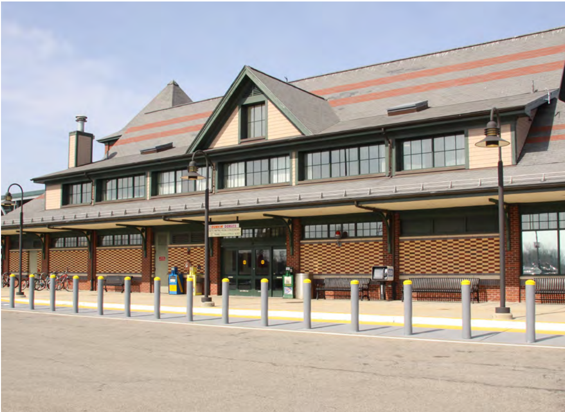
Figure 1. The James Anderson Regional Transportation Center opened at the Industri-Plex site in 2001 (Massachusetts).
