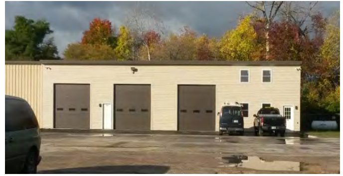
Figure 91. Kearsarge Metallurgical Corp. site (New Hampshire).
