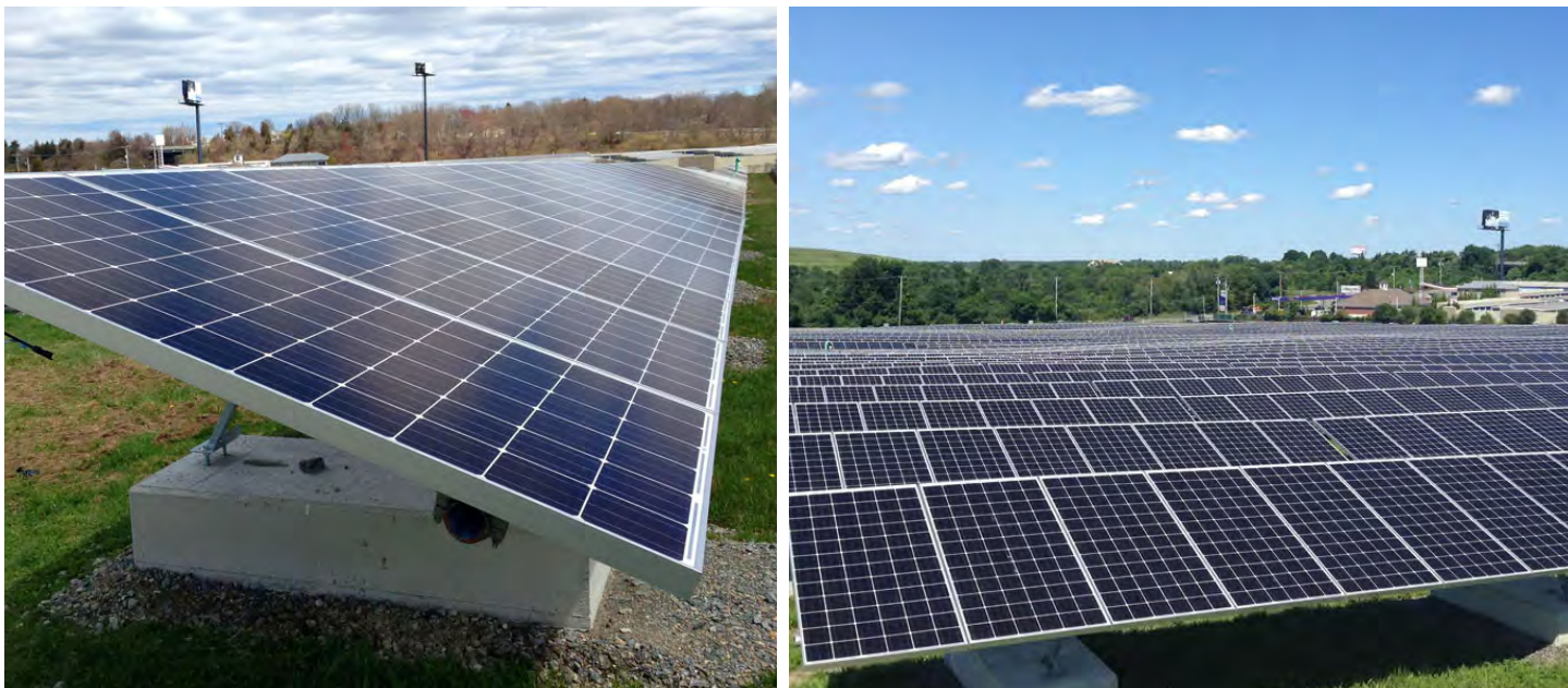
Figure 5. Over 5,000 block-mounted, fixed-tilt solar panels are in operation at the Sullivan’s Ledge site (Massachusetts).
