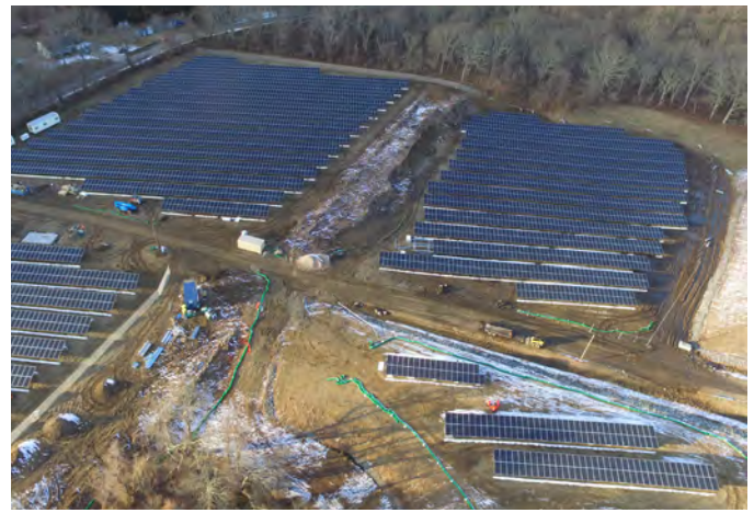
Figure 104. Aerial view of solar facility at the West Kingston Town Dump/URI site solar farms (Rhode Island). Photo used with permission of Kearsarge Energy.
