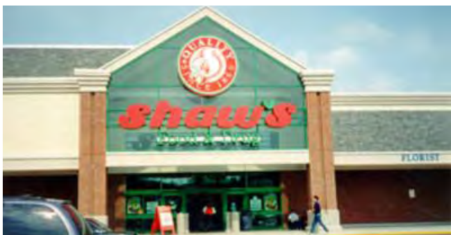
Figure 32. Reuses at the Bangor Gas Works site include a Shaw's Supermarket and Pharmacy.
