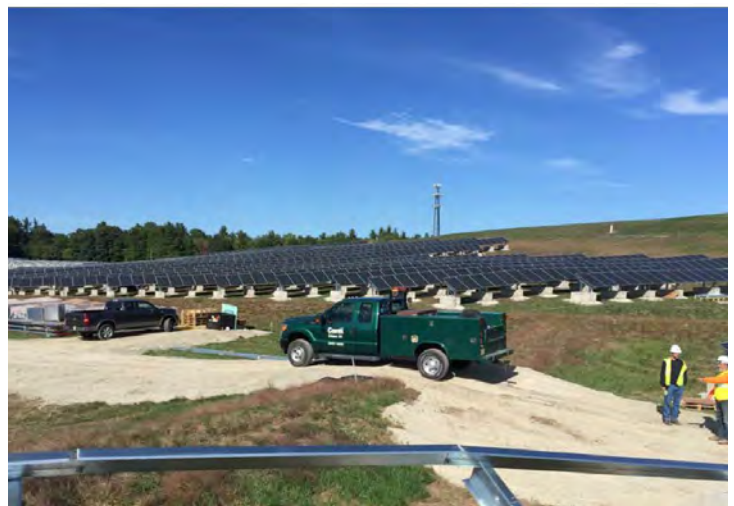
Figure 13. Installation of solar panels at the Charles-George Reclamation Trust Landfill site (Massachusetts).
