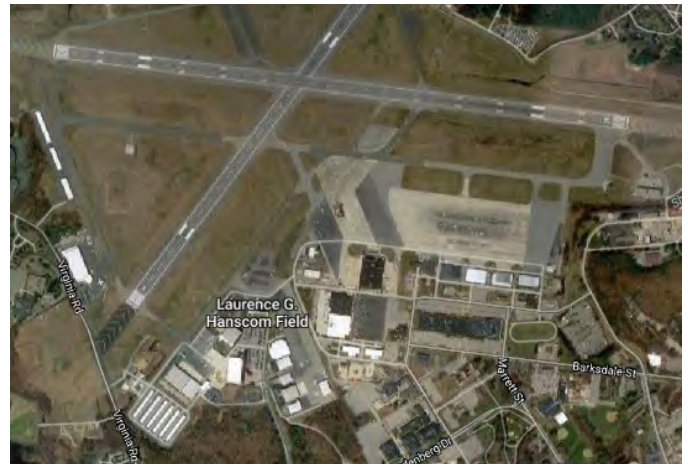
Figure 76. Hanscom Field/Hanscom Air Force Base site (Massachusetts). Imagery © 2017 Google.
