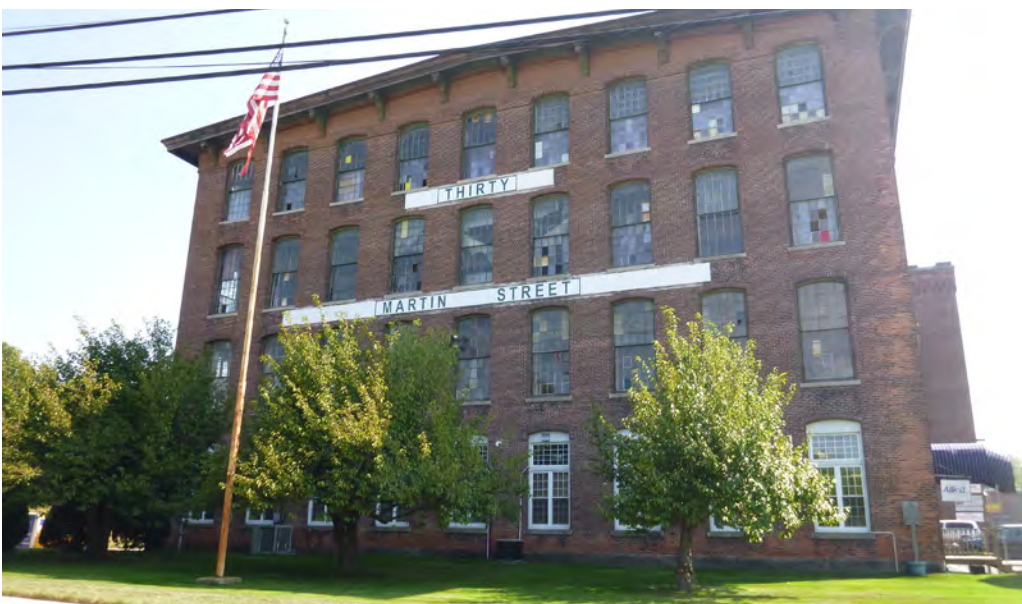
Figure 23. The 30 Martin Street building is home to several small businesses at the Peterson/Puritan, Inc. site (Rhode Island).
