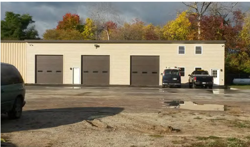
Figure 22. The former KMC building, now home to Hurteau Towing and Jon Hurteau Heating Services (New Hampshire).
