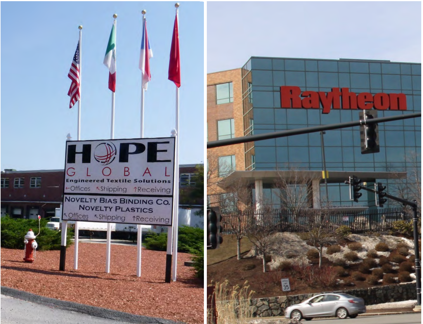
Figure 3. Left: Hope Global and Novelty Bias Binding Company develop and manufacture engineered textiles for a wide range of industries at the Peterson Puritan site (Rhode Island). Right: Raytheon facility at the Industri-Plex site (Massachusetts).
