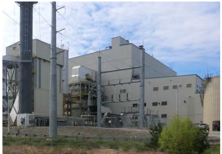
Figure 12. Biomass facility at the Gallup's Quarry site (Connecticut).
