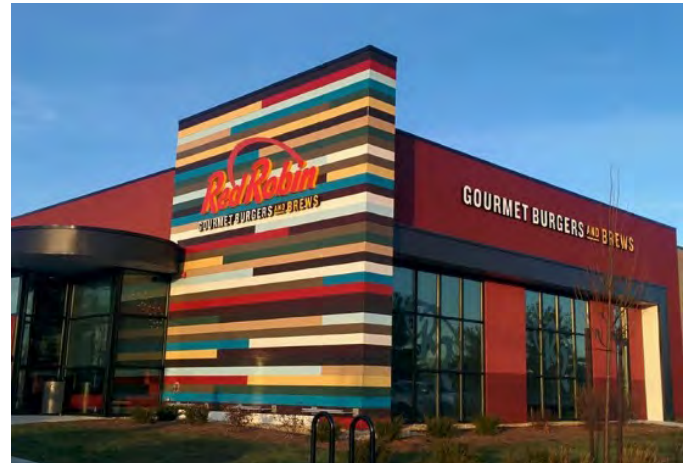
Figure 73. New restaurant at the Wells G&H site (Massachusetts).
