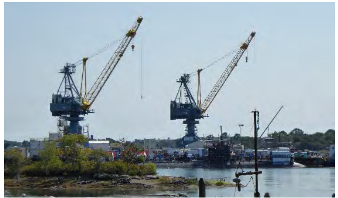
Figure 56. Portsmouth Naval Shipyard site (Maine).
