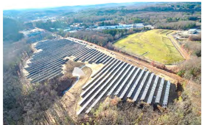
Figure 72. W.R. Grace & Co., Inc. (Acton Plant) site (Massachusetts).
