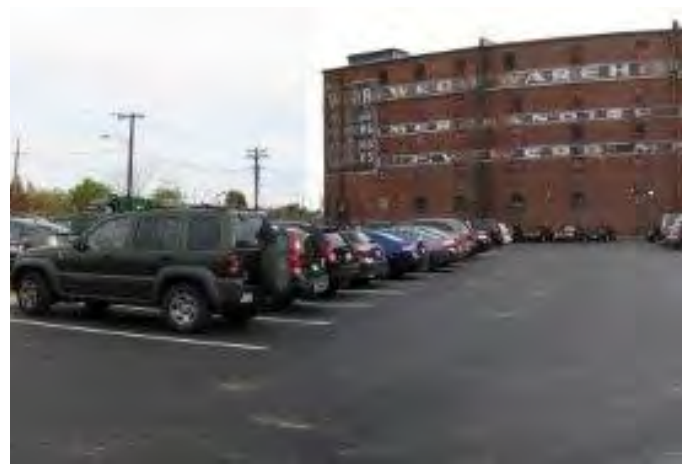
Figure 88. Universal Steel & Trading Corporation site (Massachusetts).
