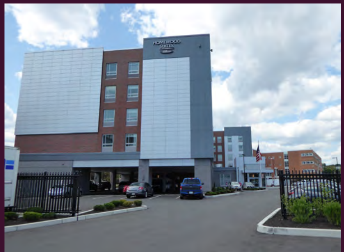
Figure 6. Homewood Suites at the Lawrence Metals (Former) site (Massachusetts).
