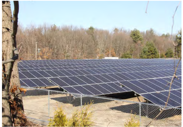
Figure 11. Completed solar panel array near the Iron Horse Park entrance (Massachusetts).
