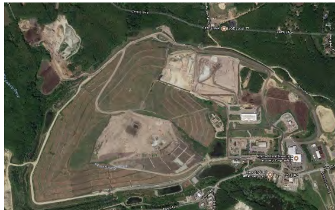
Figure 100. Central Landfill site (Rhode Island). Imagery © 2017 Google.
