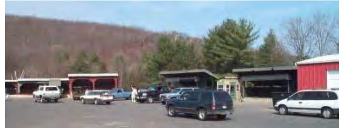
Figure 37. Barkhamsted-New Hartford Landfill site (Connecticut).
