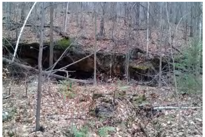
Figure 109. Former entrance to main mining shaft at Ely Copper Mine site (Vermont).
