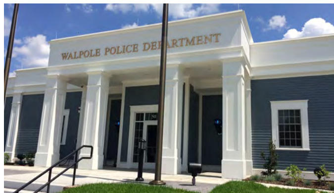
Figure 59. Police station at the Blackburn & Union Privileges site (Massachusetts).
