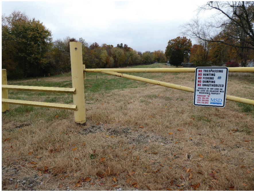
Gate and signage near the Site entrance
