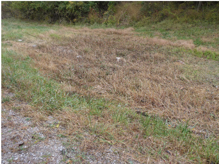
Culvert drain with vegetation on the landfill cap
