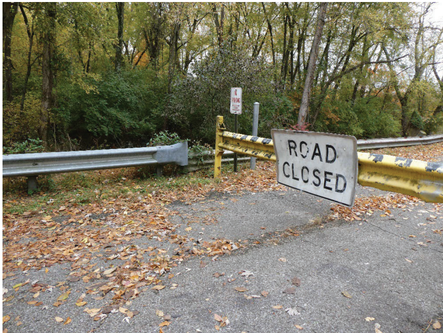
Locked gate at site entrance
