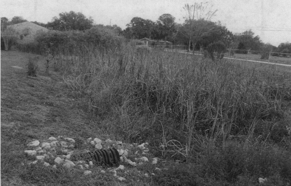
Stormwater retention pond near FFF/Landia property border.
