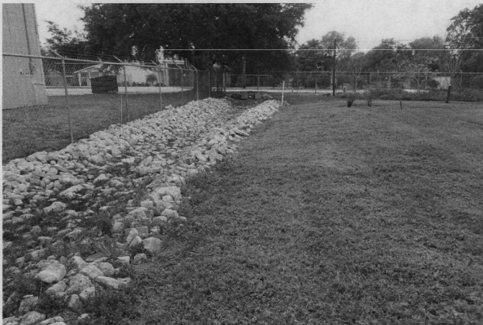
Drainage on Landia property that leads to Wayman Street Ditch.
