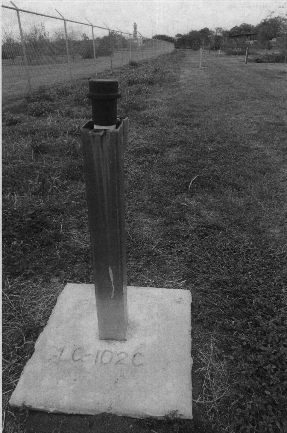
Monitoring well LC-102C on Landia property – fence between FFF and Landia properties on left.
