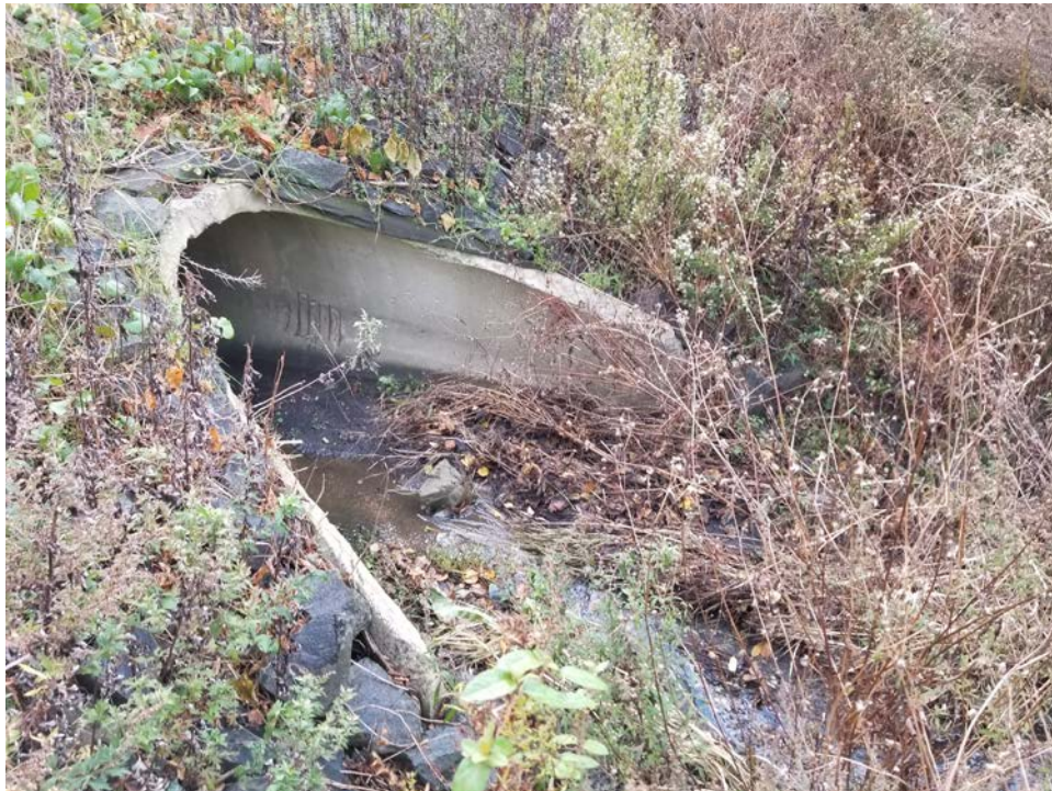
Some Siltation and Vegetative Growth – ES#1 (DS#8)
