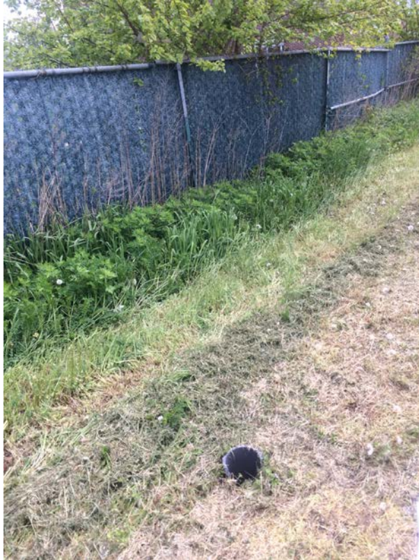
Well Casing Broken at Grade – NE-16
