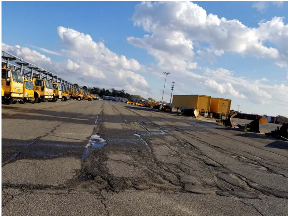
Asphalt Surface Cracks Area C
