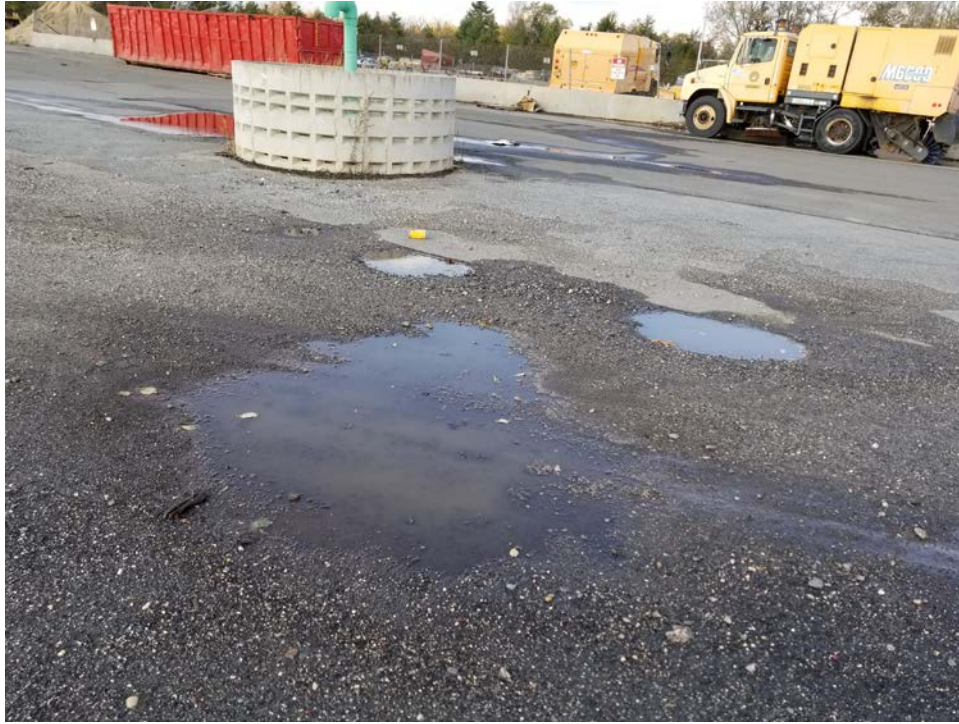
Ponding in Area A/C Border
