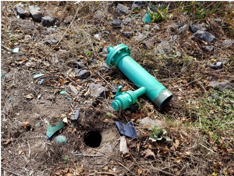
Well Casing Broken at Grade – SW-6
