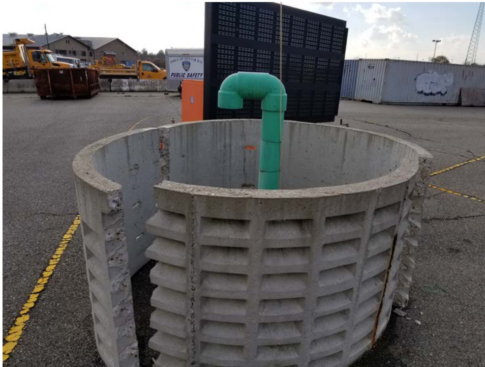
Ridge Gas Vent Well Broken Ring – R-26
