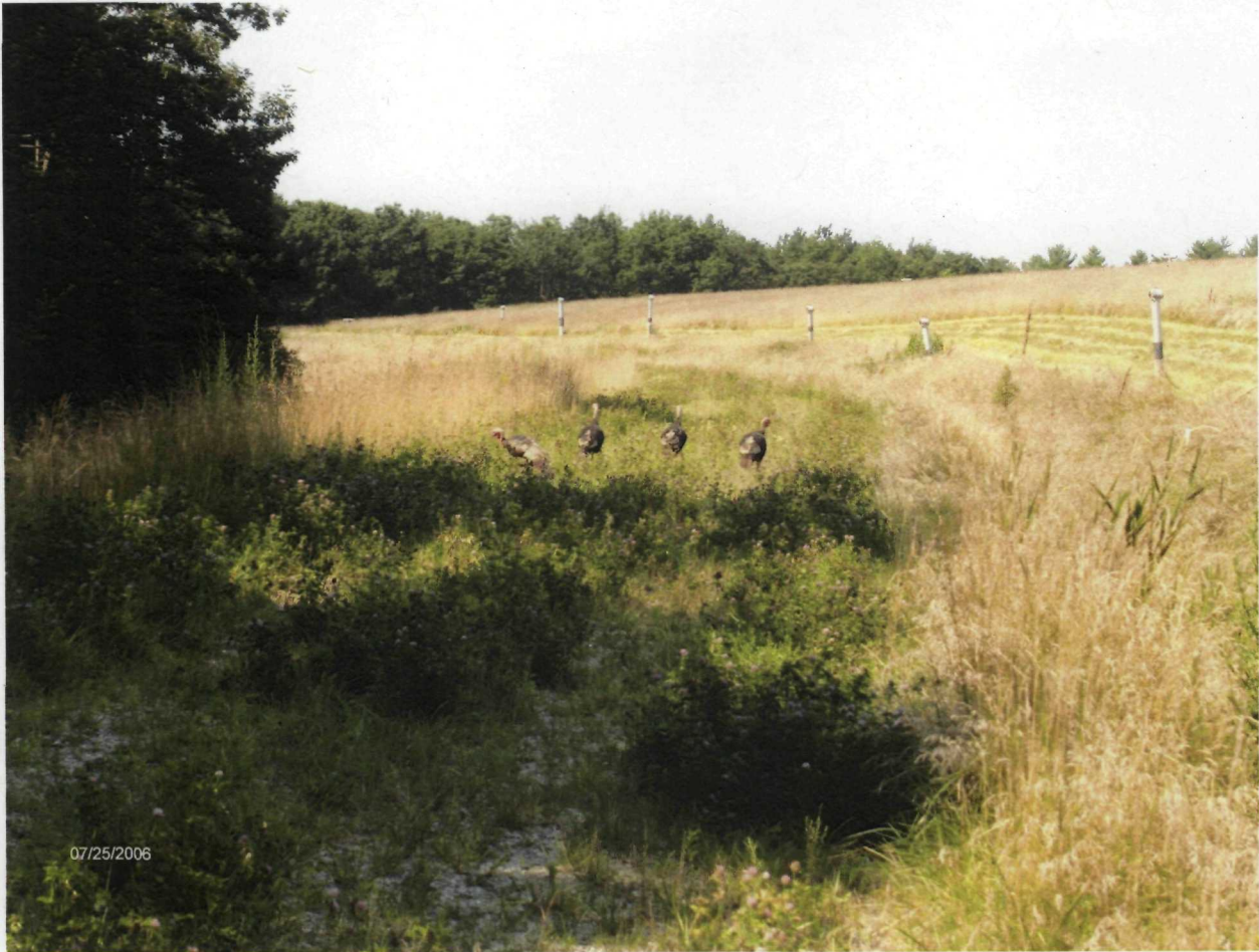
Coakley Landfill - East side
