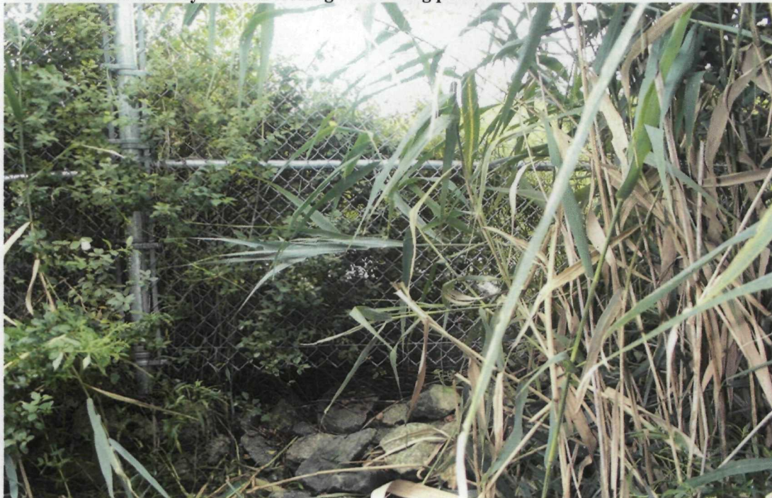
Leachate (L-1) down chute from landfill
