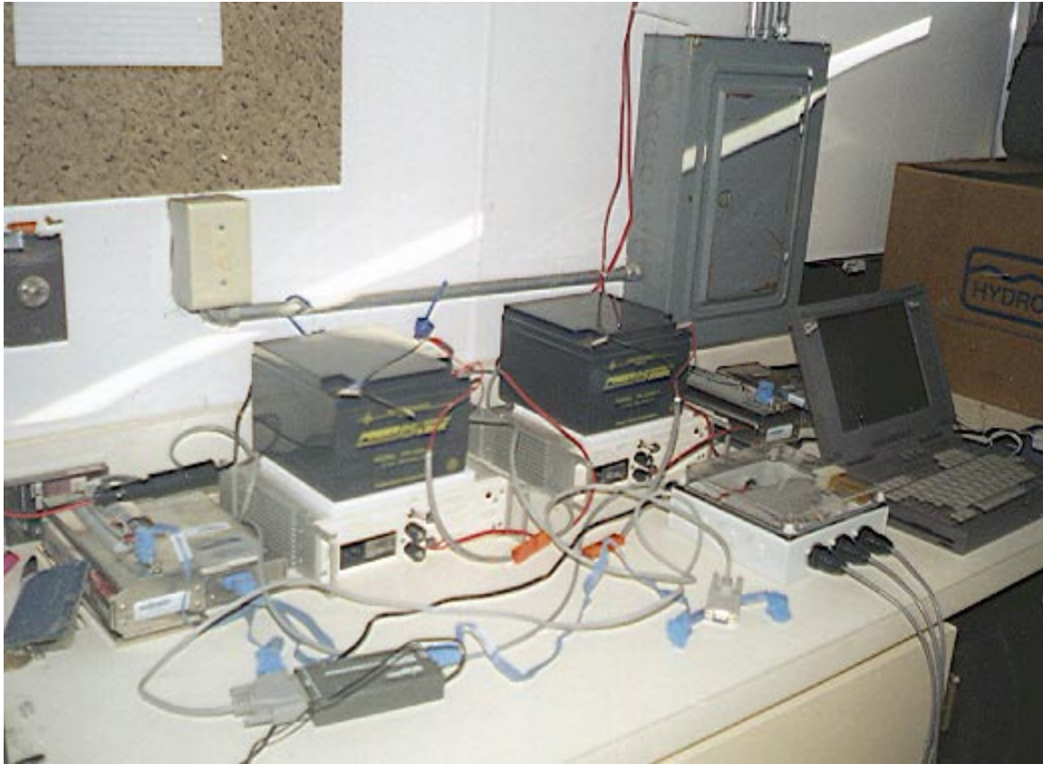
Figure 4.7. Automated data logging equipment used during the Fry Canyon barrier demonstration project.
