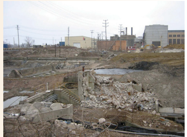
Demolition of existing infrastructure and buildings
