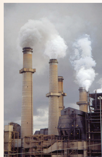
Four Corners Power Plant
