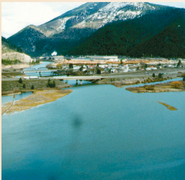
Milltown Reservoir, looking up towards the Blackfoot River
