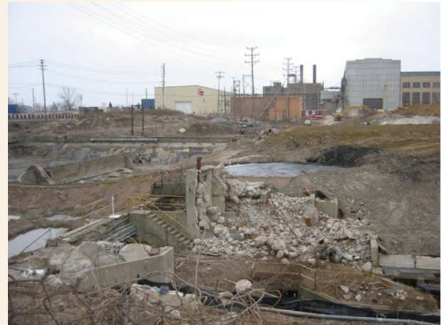
Demolition of existing infrastructure and buildings
