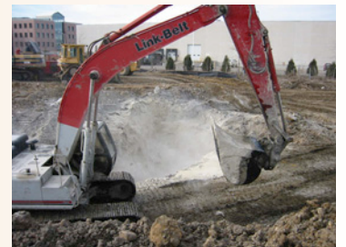
Sediment stabilization mixing operation
