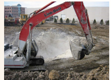
Sediment stabilization mixing operation
