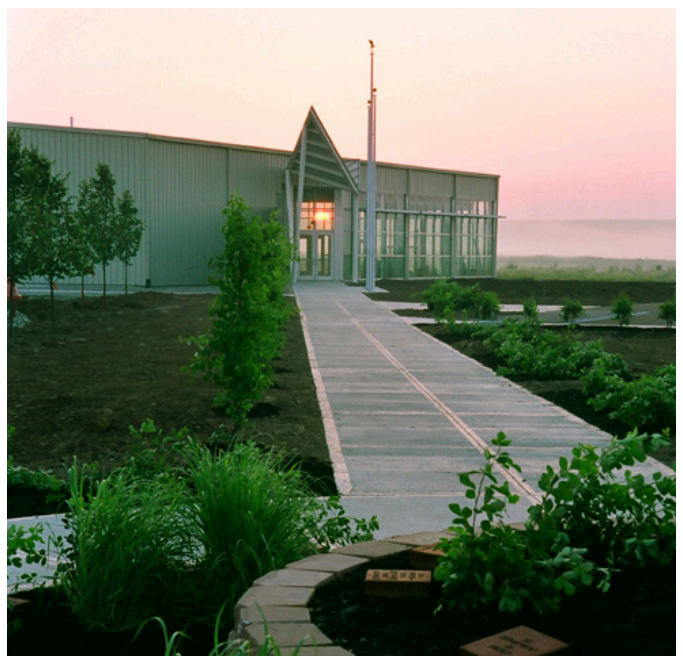
The site's warehouse prior to renovation (left), during renovation (above top) and in adaptive reuse as the Fernald Preserve visitor center (above bottom). Source: glaserworks architecture
