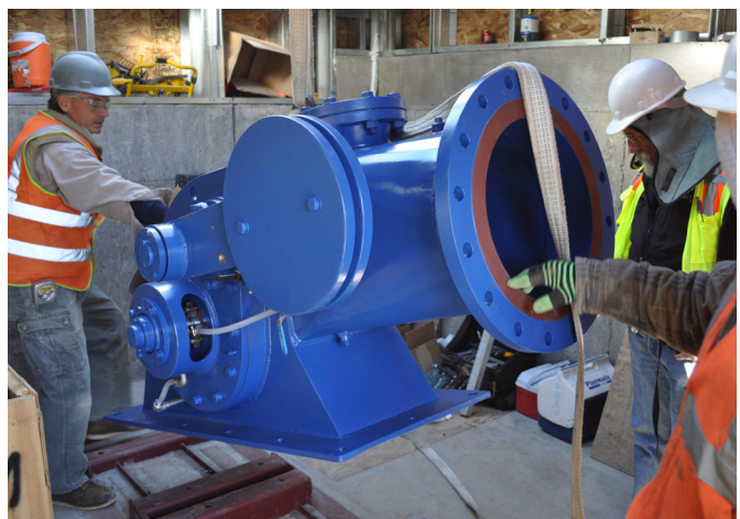
Installation of hydroelectric equipment at the Summitville Mine site in Colorado in 2010. Source: EPA
