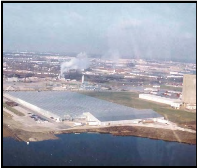
Aerial View of Greenhouse
