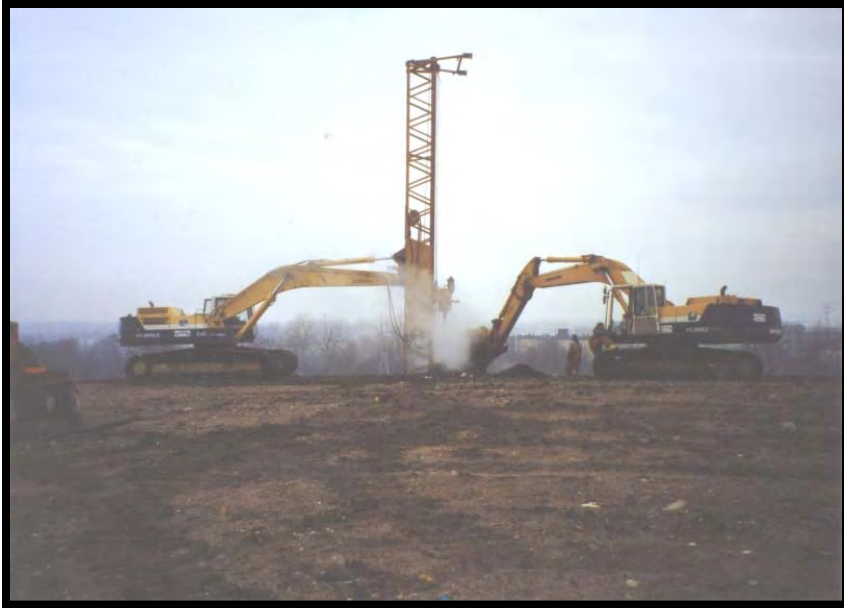
Well Drilling at South Side
