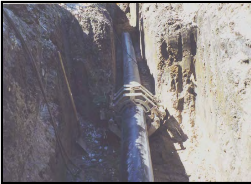
Pipeline to Rolls Royce 7200 ft. 12 inch HDPE
