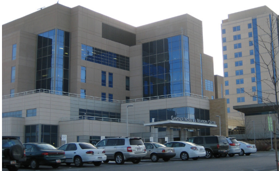
A side view of the Intermountain Medical Center at the Murray Smelter Superfund site.
