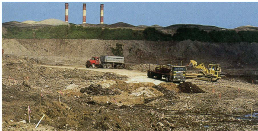
At the Harbor International Golf Center in Chicago, fairways, greens, and bunkers were crafted with the use of wastewater biosolids blended with other locally available materials, to form a contoured golf course out of the previously flat topography.
