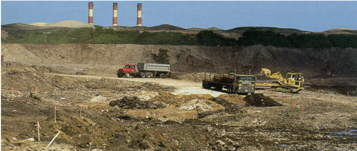
Construction of the Harbor International Golf Center
