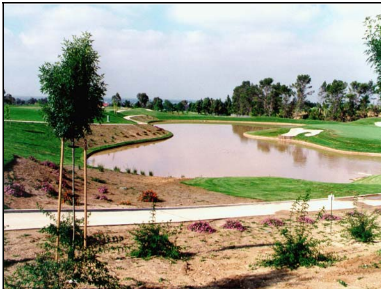
At the McColl site, designers included landscaped areas as part of a golf course built over a cover system. Designers omitted a layer of cobbles for covers over landscaped areas to minimize settlement caused by the weight of the cap.
