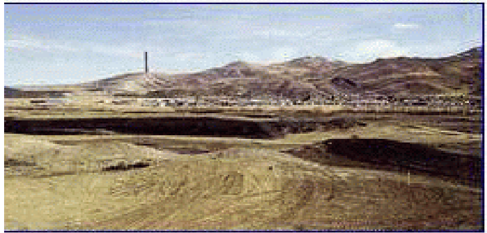
Anaconda site at the early stages of the remediation
