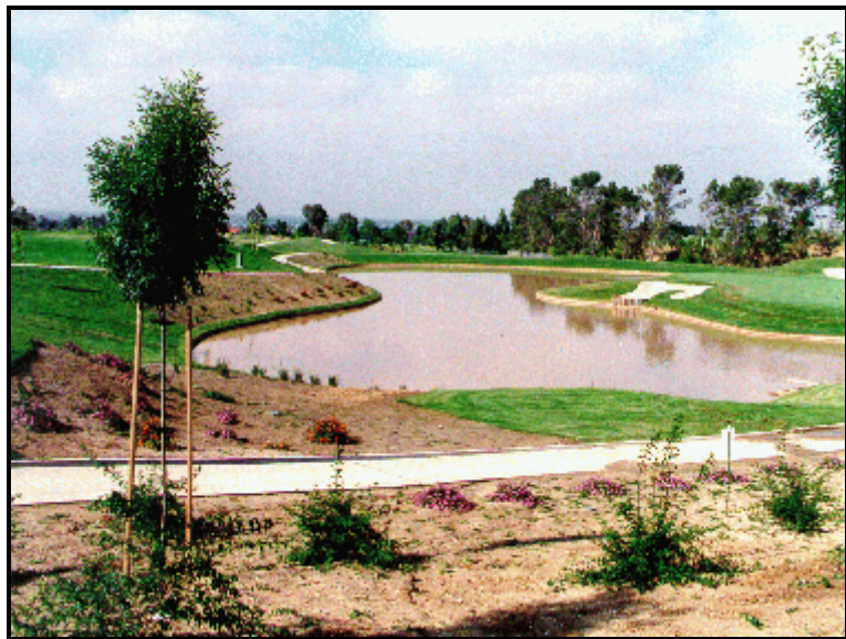
At the McColl Superfund site in Fullerton, California, designers included landscaped areas as part of a golf course built over a cover system. Designers omitted a layer of cobbles for covers over landscaped areas to minimize settlement caused by the weight of the cap, using institutional controls instead.
