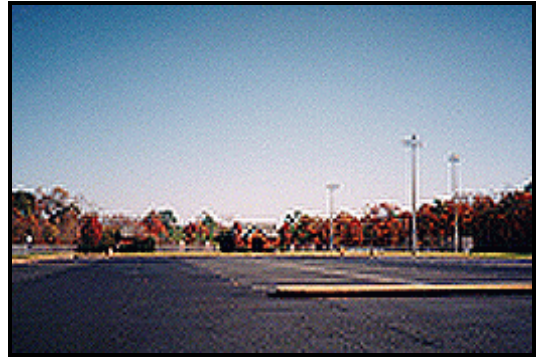
A parking lot for the sports fields at the Chisman Creek site in Yorktown, Virginia, was built over a portion of the cover system.
