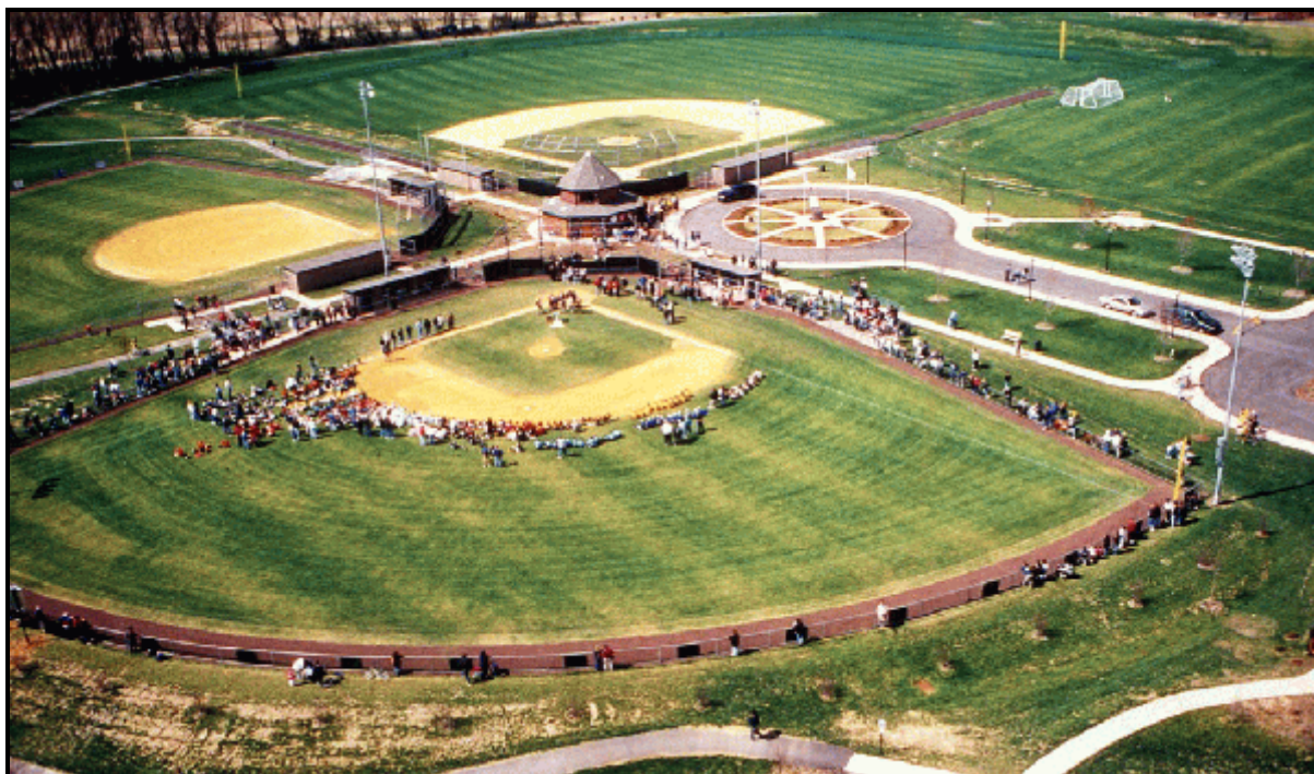
A sports complex, including six baseball and soccer fields, were built over waste containment areas at the Lapari Landfill Superfund site in Mantua Township, New Jersey.
