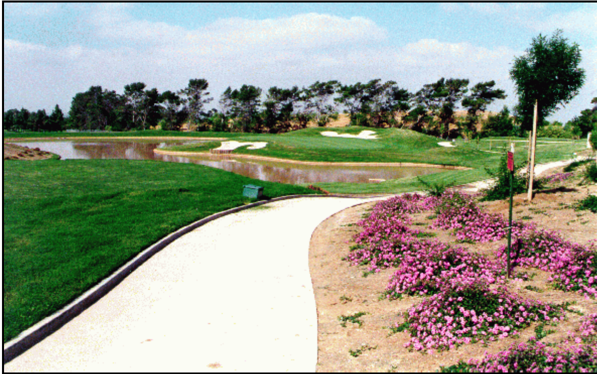
At the McColl Superfund site in Fullerton, California, a geogrid-reinforced cap was used to prevent depressions resulting from settlement. This former refinery waste dumping ground is now being used to extend an existing golf course.
