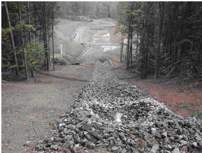
Figure 2-3. Constructed Wetland for AMD Treatment, Dents Run Watershed, Pennsylvania
