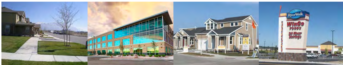
Residential and commercial development at Bingham Junction, 2011.
