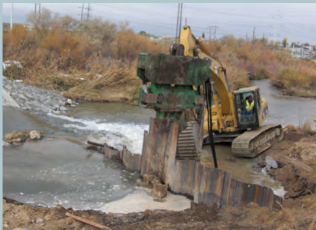
Before: The sheet pile dam across the Jordan River was damaged and needed to be removed. The failure of the dam could have allowed river water to erode the riverbank, releasing capped site contaminants.
