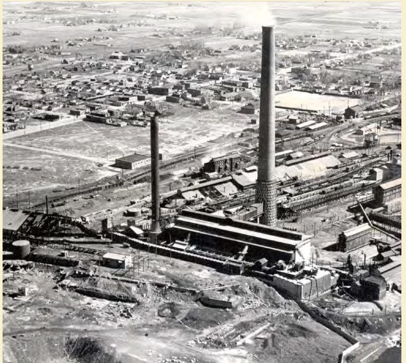
Smelter facilities at the Midvale Slag site, 1941
