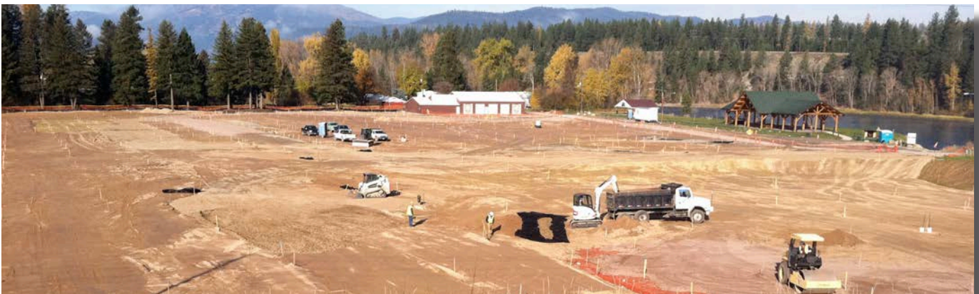
Backfilling and site grading
