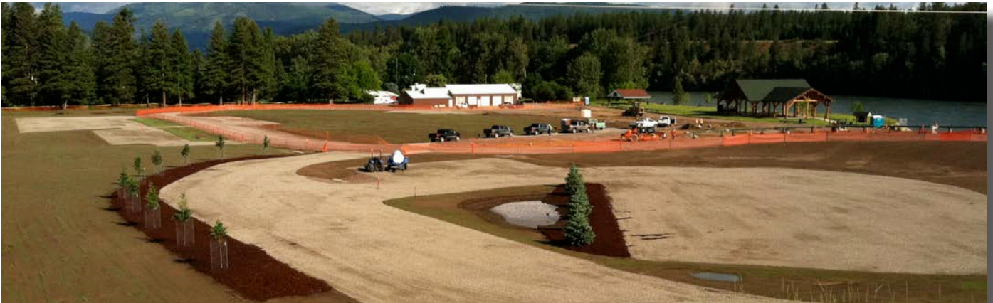
Revegetation, stormwater management, roadbed installation
