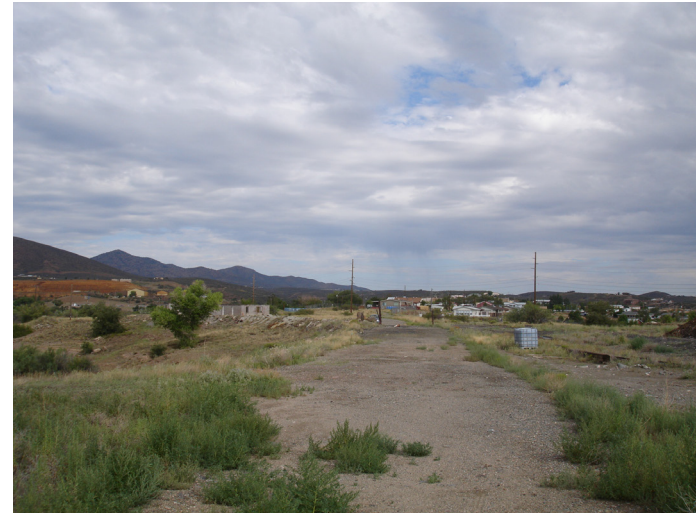
Primary access road connects the Smelter area to downtown Dewey-Humboldt
