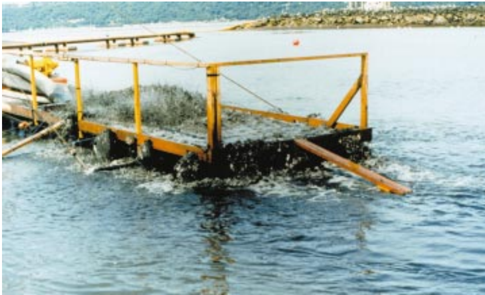
Figure 7. Spreader box or “sand box” for hydraulic pipeline discharge
