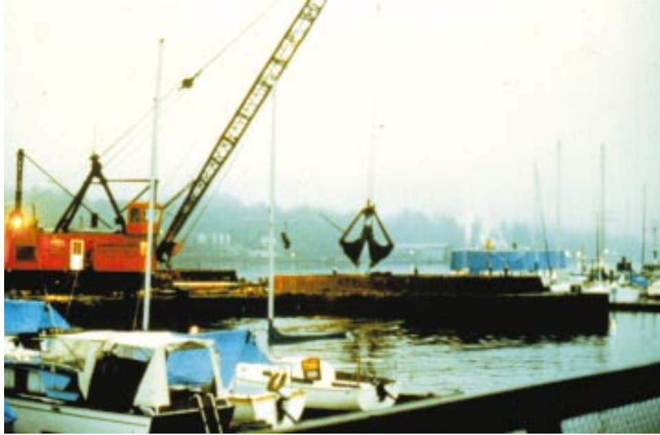
Figure 35. One Tree Island Marina project
